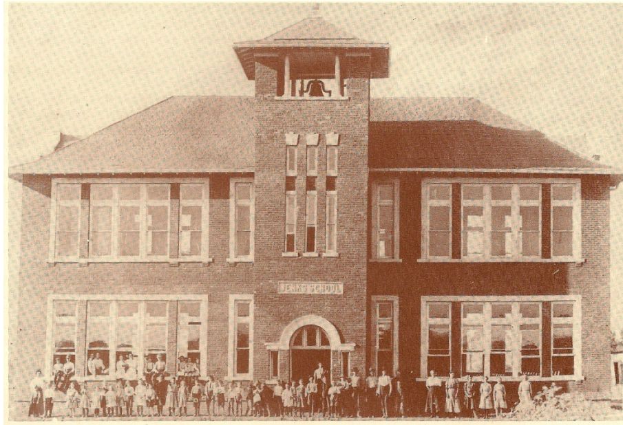
Figure 3 First Jenks Public School Building, 1908
