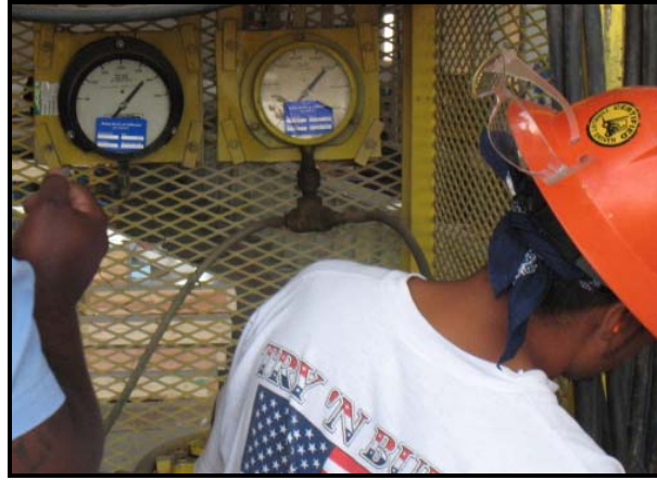
(b) Monitoring the gauge pressure of the jack
