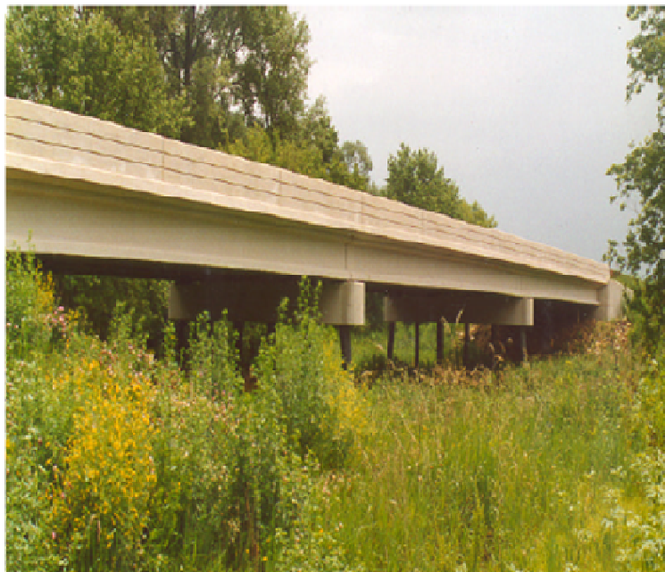
Figure 7.1: Concrete IAB (Photo Courtesy of Huang et al. 2004)
