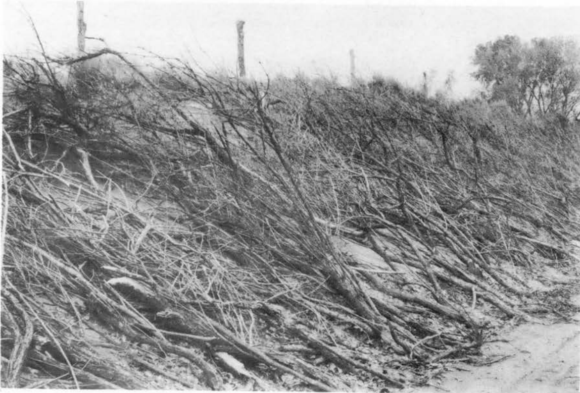
Figure 25.--Brush rip-rap for wind erosion control and quail cover along a sandy road shoulder, Gene Howe Game Management Area, Texas Game and Fish Commission, two miles north, six miles east of Canadian, Texas, May 7, 1957.
