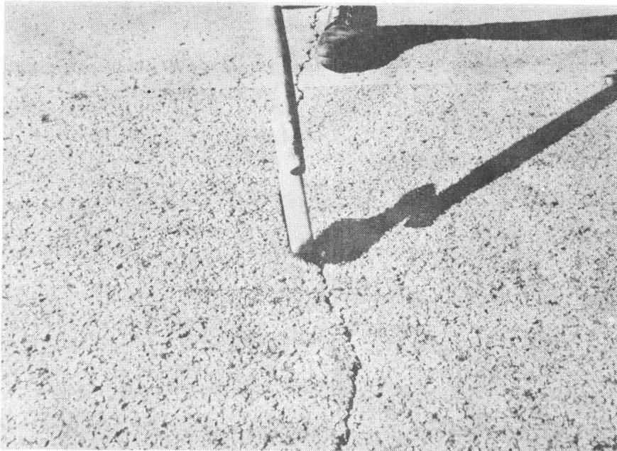
Figure 4. Wire Brushing a Traverse Crack
