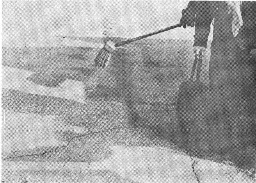
Figure 7. Installing and Sanding Emulsion Sealants
