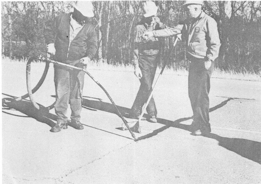
Figure 6. Installing High Viscosity Sealants
