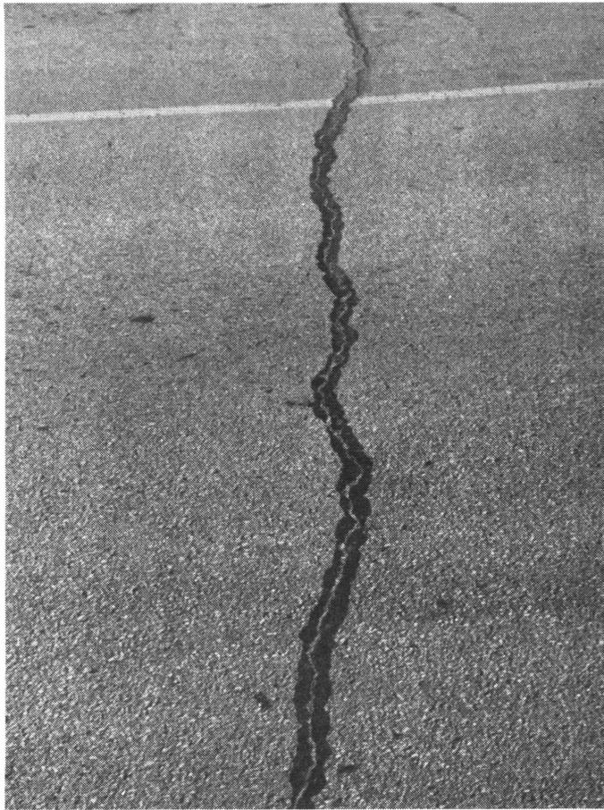
Figure 17. Cohesive Failure in CRS-2 Sealed Crack
