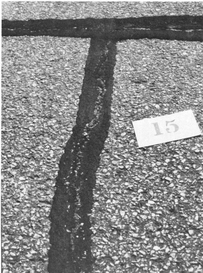
Figure 22. Adhesive and Cohesive Failures
