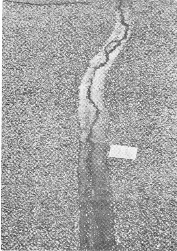
Figure 12. Cohesive Failure in Asphalt
