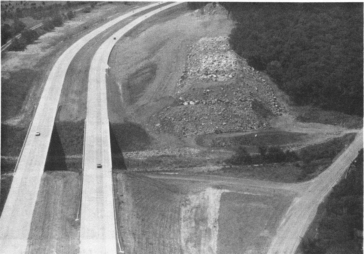
Figure 30. Limestone Creek and US 69 Looking South, 1988
