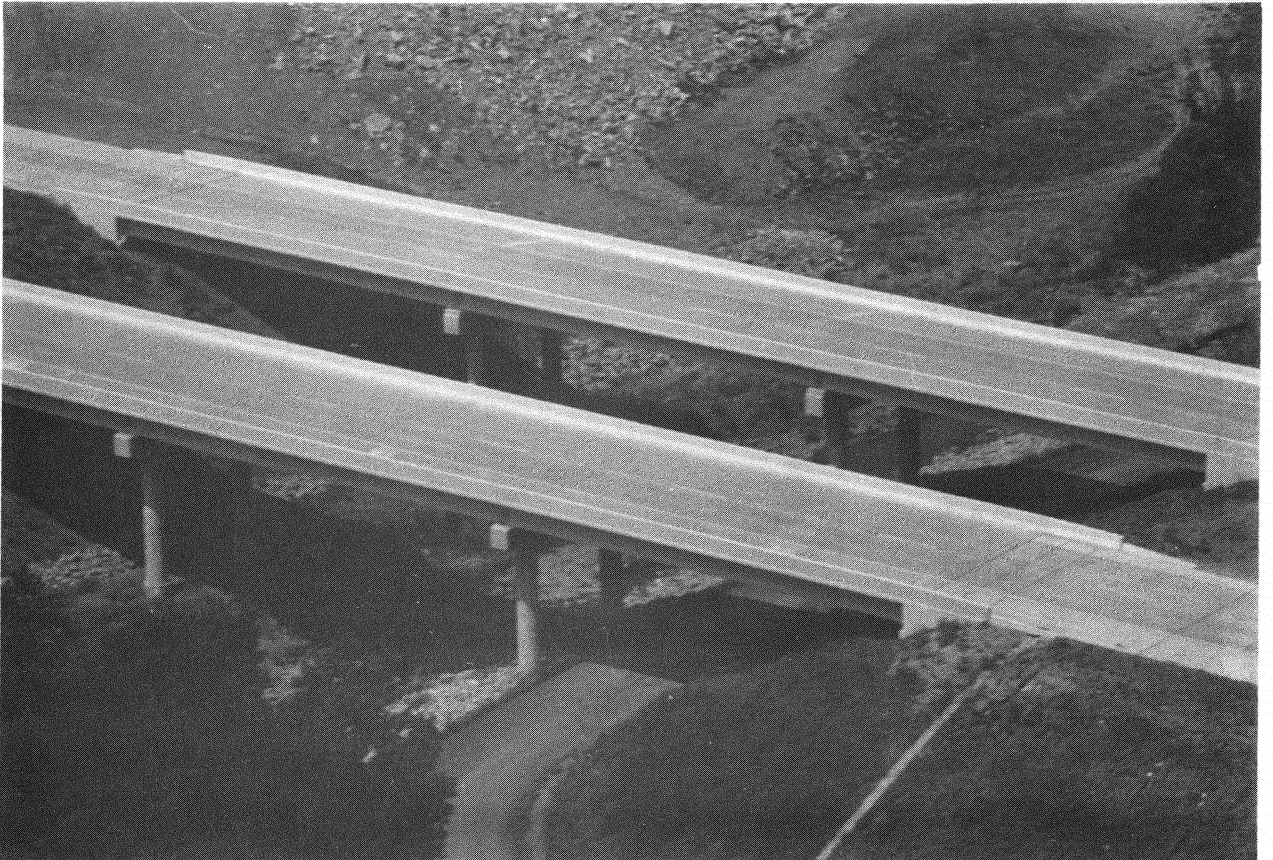
Figure 29. Completed New Twin Bridges at Limestone Gap
