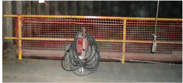
Figure 11. Sweep auger worker protection fencing.
