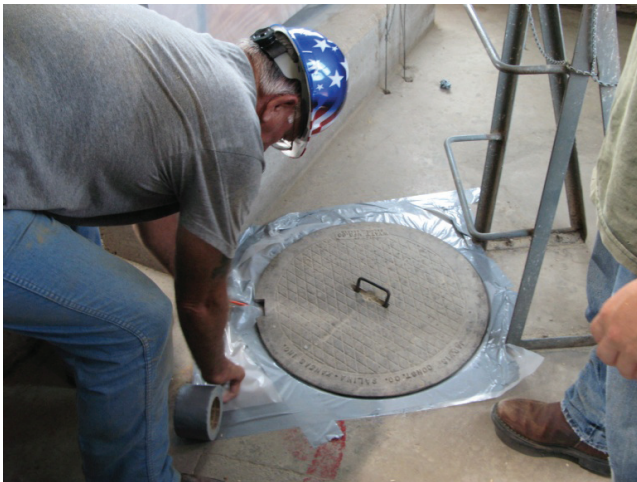
Figure 19. Sealing manhole cover with polyethylene film in a concrete elevator.
