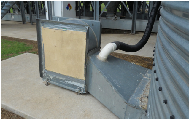
Figure 18. Aeration fan intake sealed with polyethylene film and duct tape. A plywood support panel is secured over the fan opening to protect the polyethylene film from wind damage.
