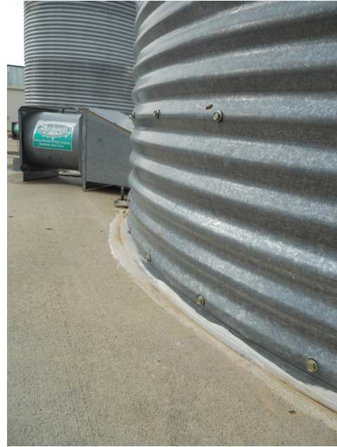
Figure 12. Base of bin sealed with elastomeric sealant.
