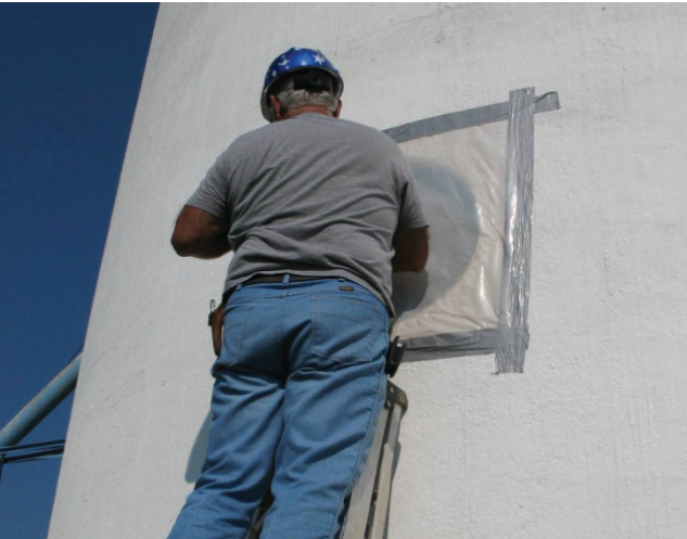
Figure 16. Temporary sealing of hatch on concrete silo prior to fumigation.
