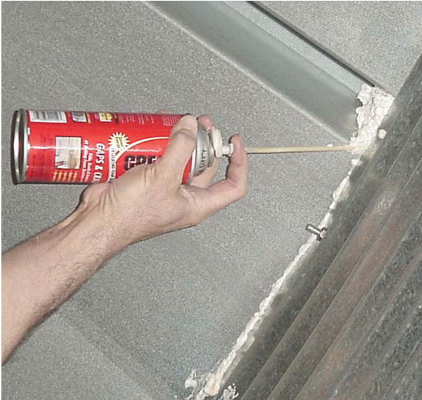
Figure 9. Bin roof and sidewall seam sealed with silicone caulk and closed cell foam.
