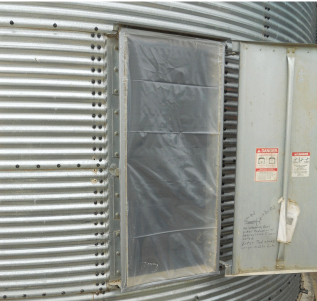
Figure 17. Access door sealed with polyethylene film and duct tape.
