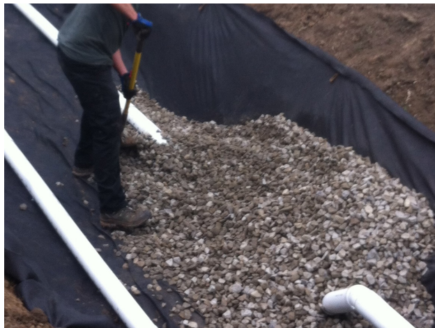
Figure 5. Installation of an underdrain.
