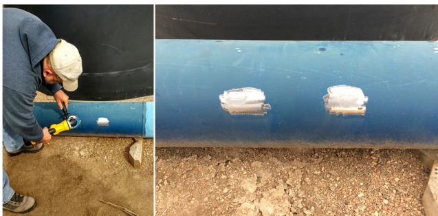
Figure 9. Pipe surface preparation for flow measurement in the field.
