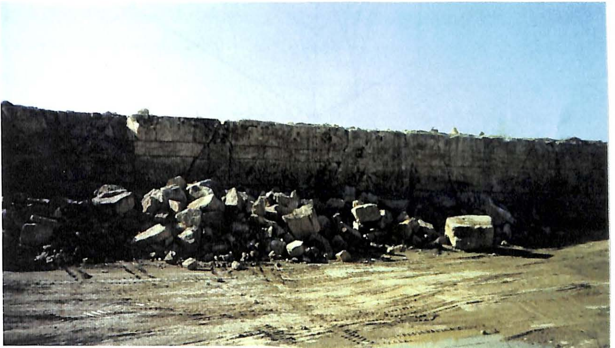
Figure 19. A. Photograph of a fracture zone in the north wall of the quarry.
