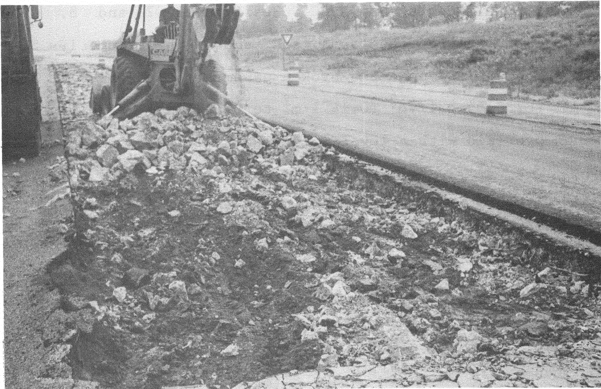
Figure 7. Soft subgrade sections were removed and replaced with AC.
