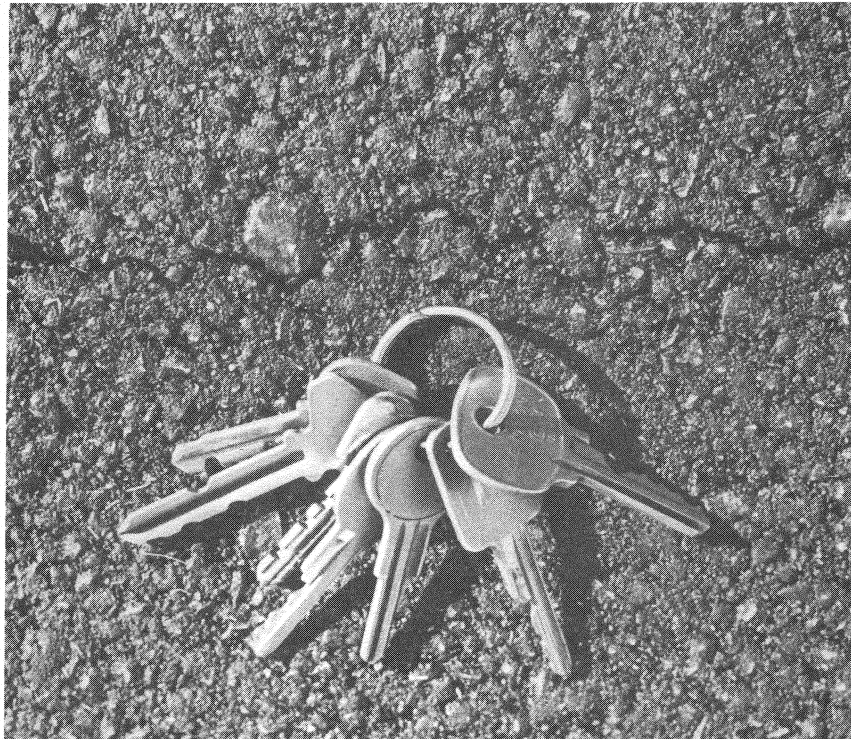
Figure 14. Close view of transverse crack over joint in Petrotac treated section - overlay less than 1 in. thick.
