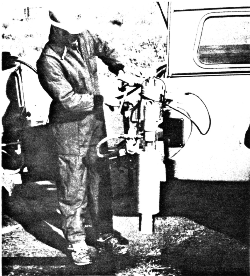
Figure 25. Core samples were taken from the deck.
