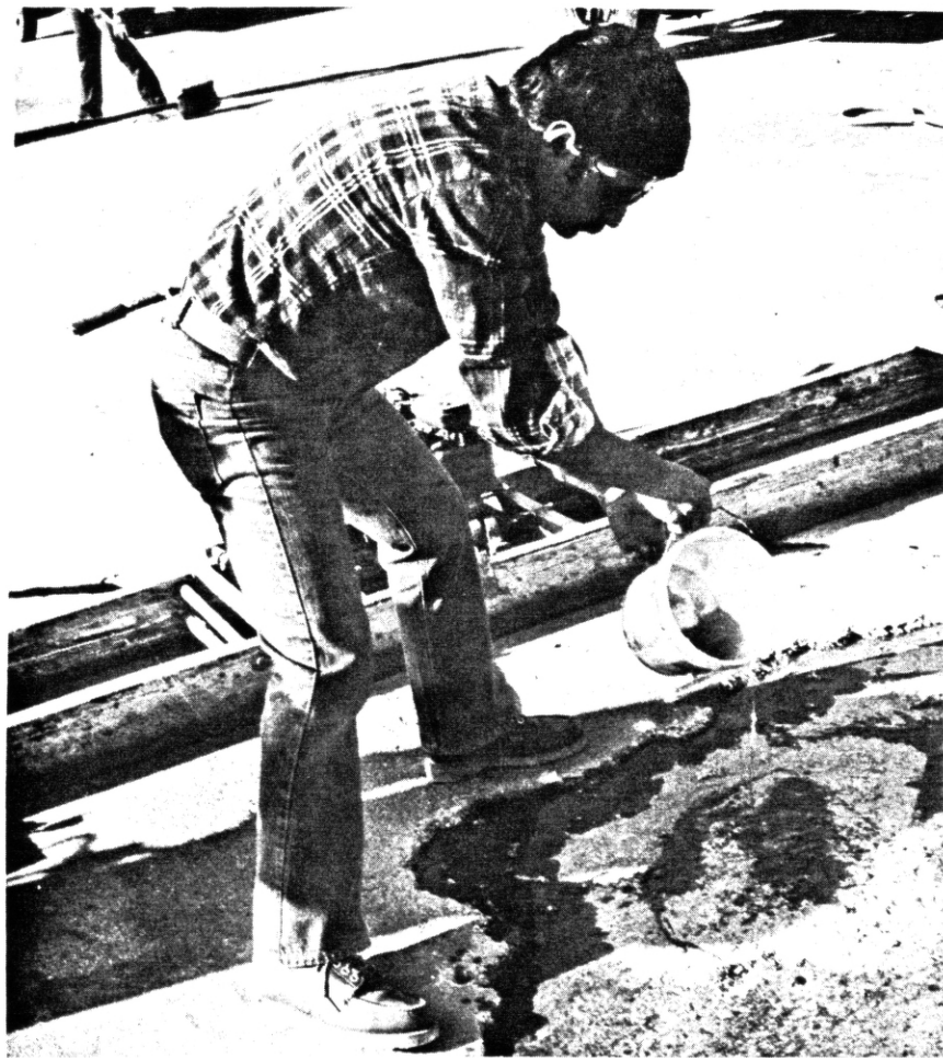
Figure 23. Delaminations were generously tackcoated.
