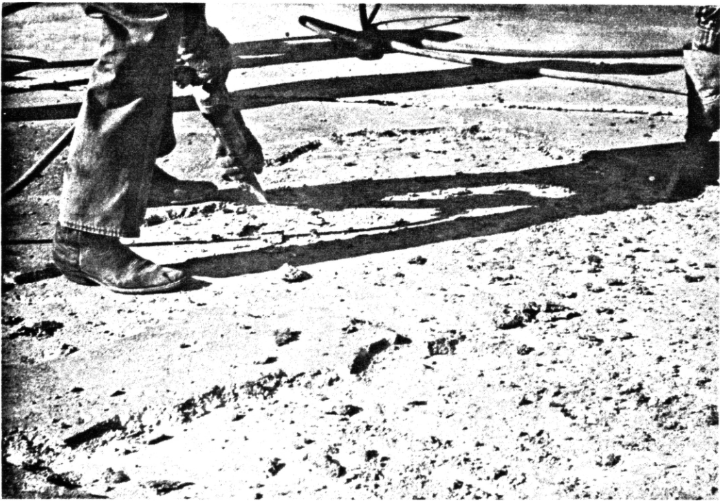
Figure 21. Unsound polymer concrete was jackhammered away.
