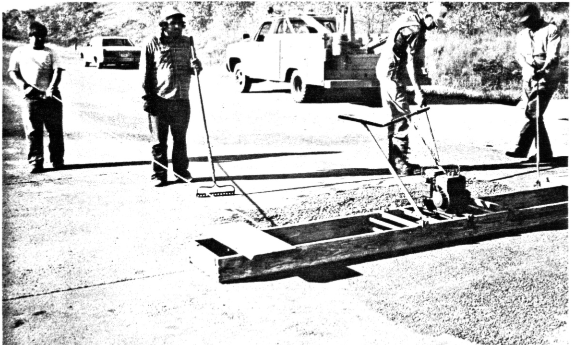
Figure 24. A shopbuilt screed compacted the patches.
