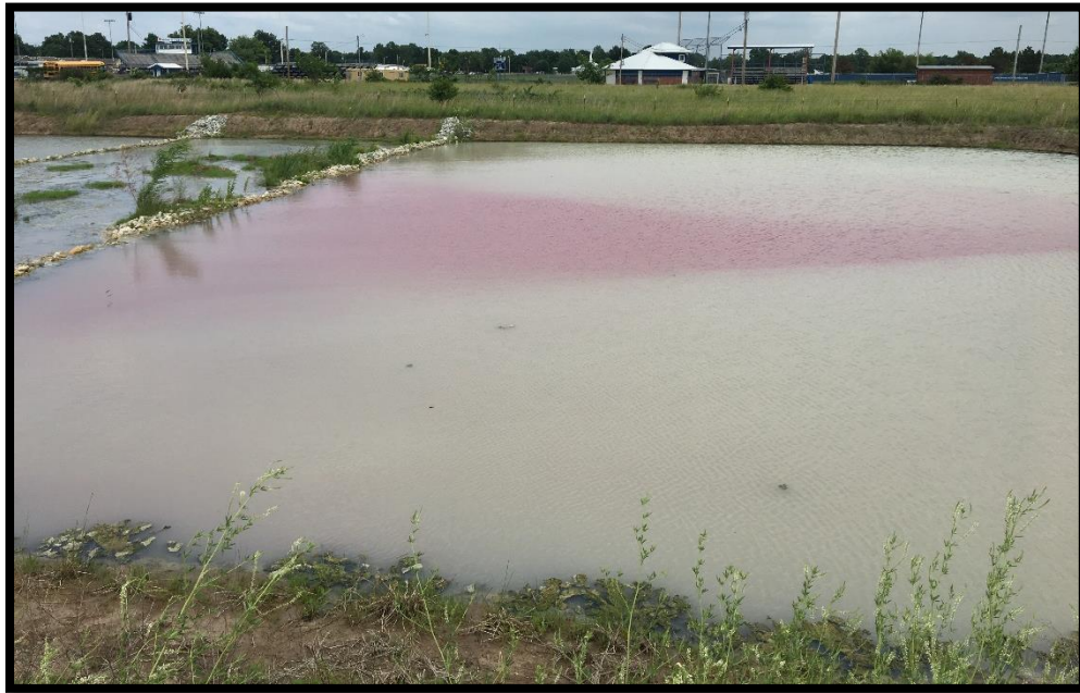
Figure 5.3. Purple sulfide oxidizing bacteria seen in Final Polishing Unit (FPU) in June 2018
