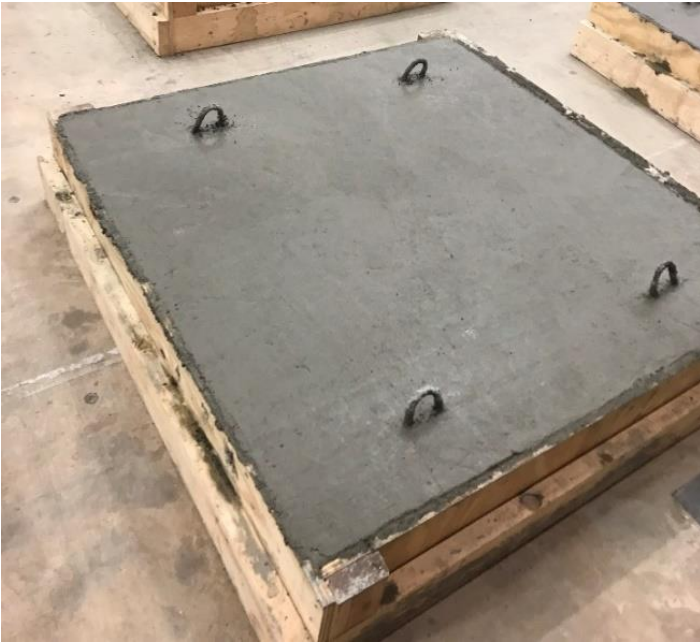
Figure 10: Panel immediately after casting
