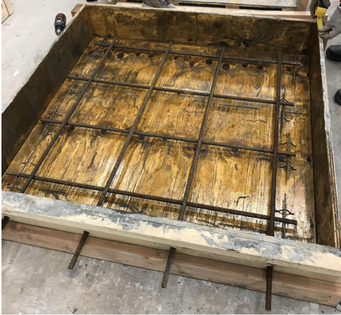
Figure 9: Rebar layout prior to casting
