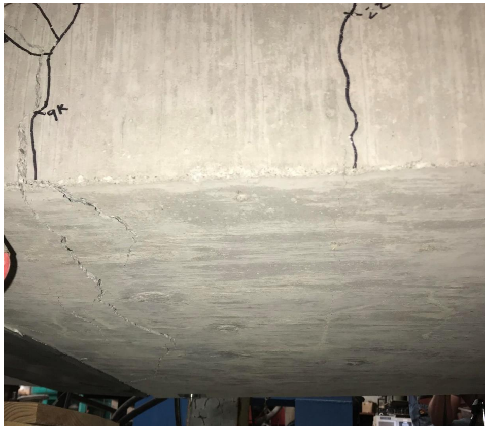
Figure 54: Cracks formed underneath load point on slab 2
