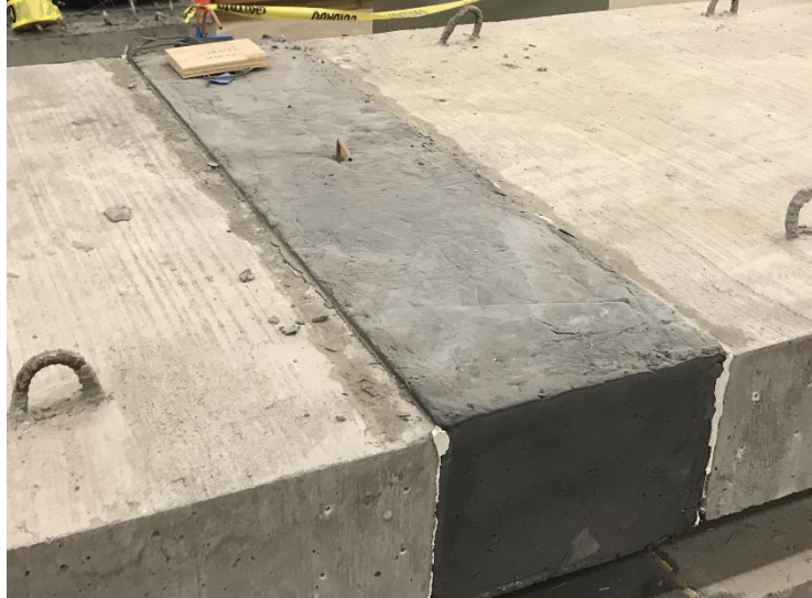
Figure 14: UHPC joint after curing
