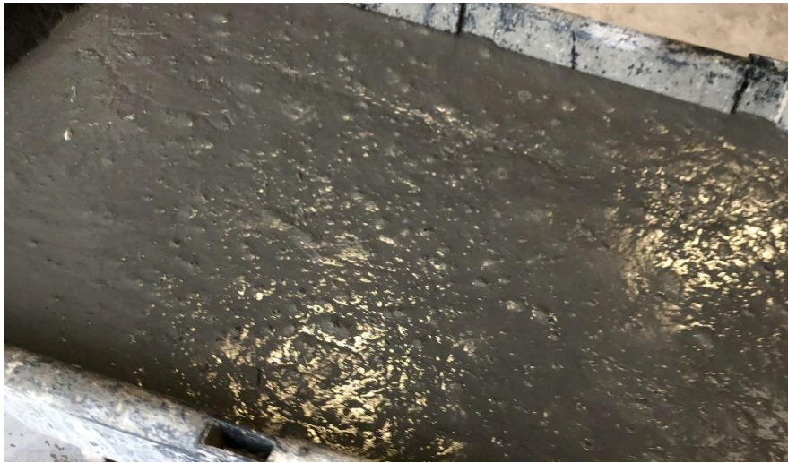
Figure 31: Modified J3 UHPC after mixing
