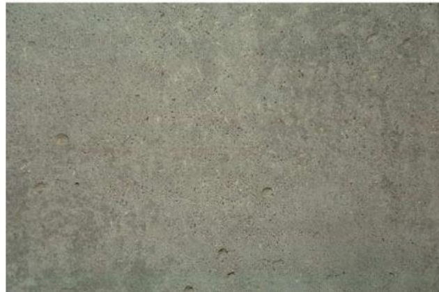
Figure 2: Steel Brushed Surface Preparation (Julio et al. 2004)
