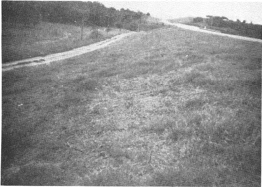
A weed infested area in Division 4, west of Cushing, on SH-33 before weed control treatments (top photo). Bottom photo shows the same area one year later after being treated with atrazine, 2,4-D and DSMA to control the unwanted weeds.
