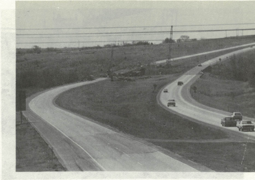
Figure 1: The project site is located on the northbound lanes of the Cow Creek Bridge on I-35 south of Perry, Oklahoma.
