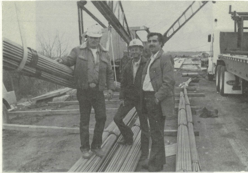
Figure 5: Carefully guiding bundled rebars to the wooden beams.
