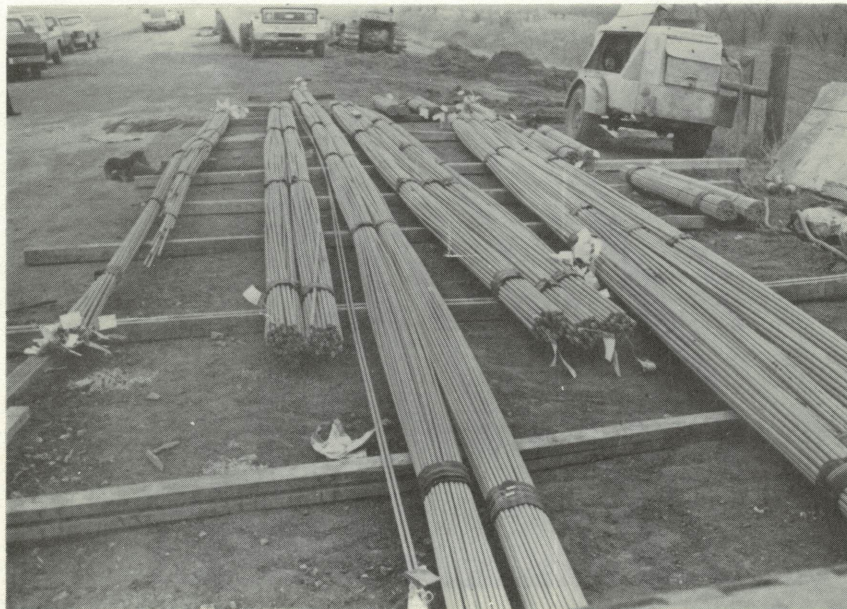
Figure 6: Coated rebar bundles were shipped and stored on wooden 2 x 4's.
