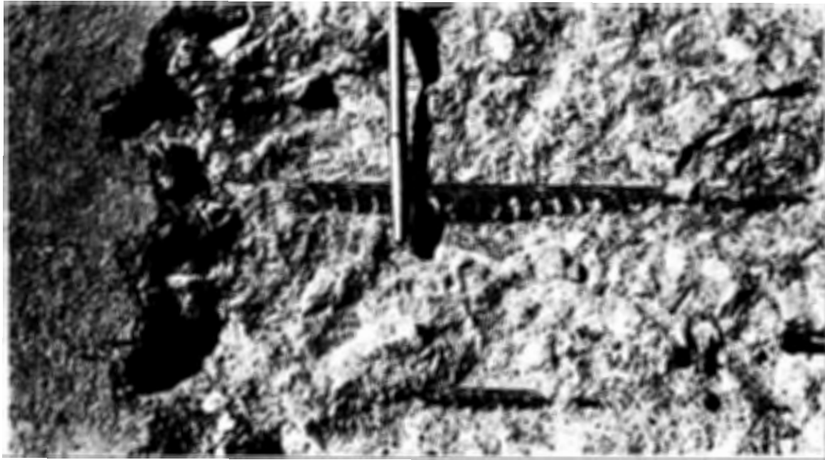
Photograph 7: The bottom course was placed to 0-1/2 inch above the reinforcing bars.
