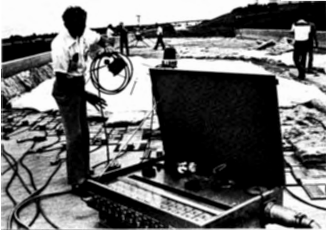
Photographs 21 & 22: Blankets and insulation were placed and covered with mesh netting and weights to prevent wind disturbance. Portable flood lights were used for night operations.
