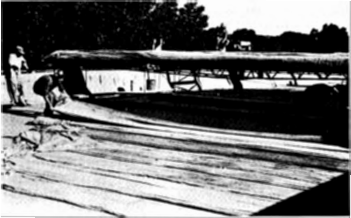
Photograph 9: The wax bead concrete overlay was placed and finished 28 days after the bottom course.
