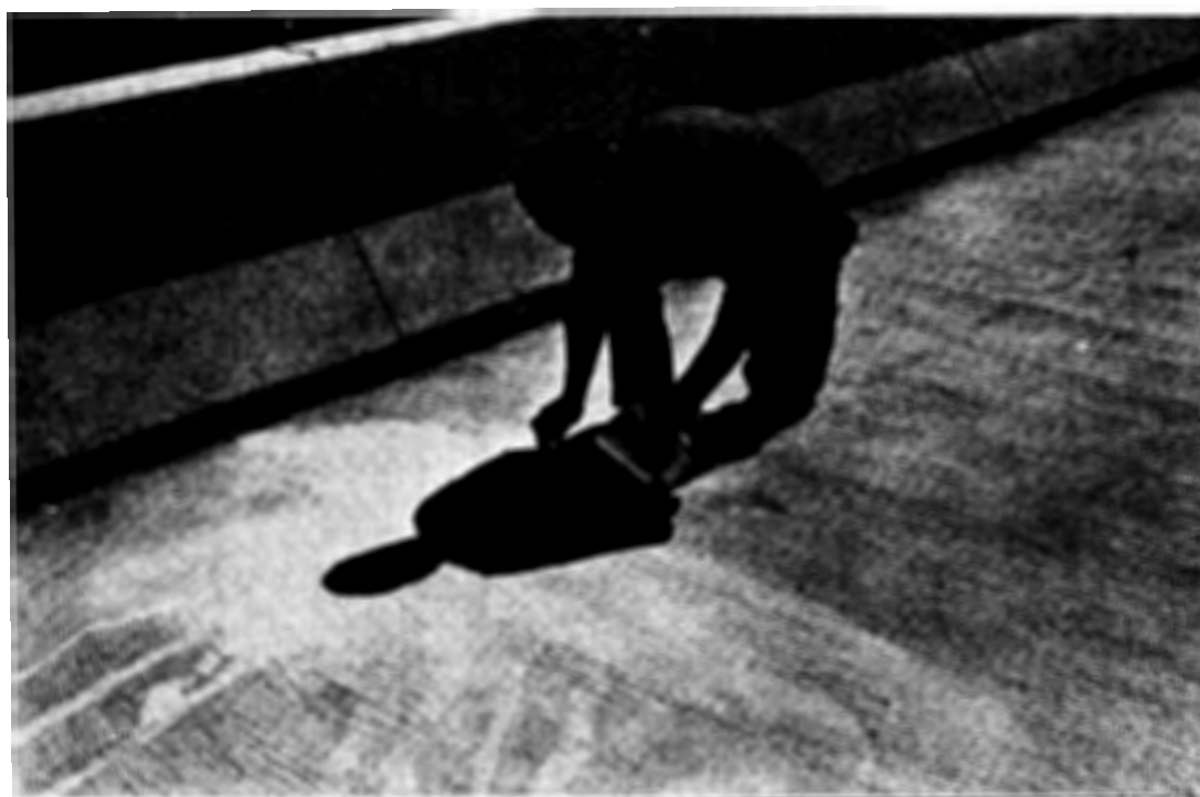
Photographs 27 & 28: Several cores were taken from the deck to determine the sealing effectiveness after heating. The holes were patched and sealed.
