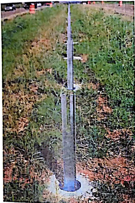
Fig. 5a: Posts and base caps in position ready for cable placement.
