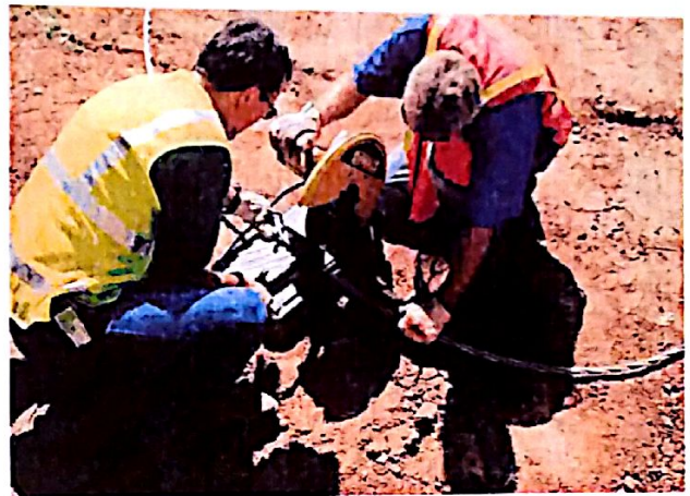
Fig. 5b: Cutting cable for end fitting.
