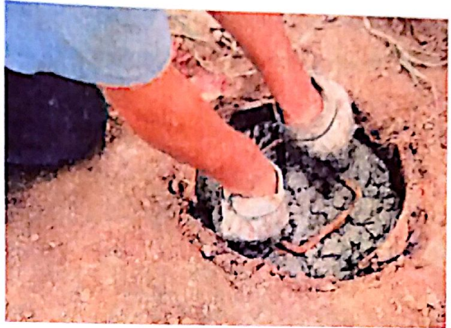
Fig. 4b: Placing reinforcing steel into base.
