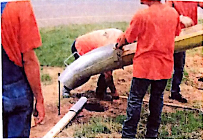
Fig. 4a: Placing concrete for post bases.
