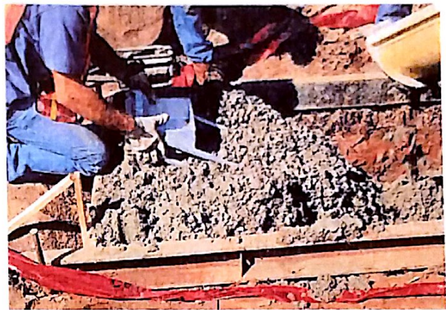
Fig 1b: Placement of anchor plate in fresh concrete.
