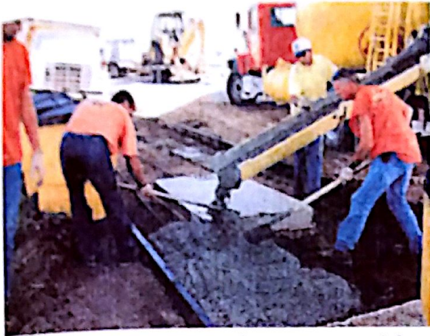
Fig. 2a: Placing concrete for attenuator slab.
