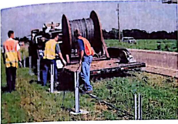
Fig. 5g: Placing bottom cable into posts.
