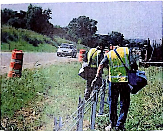
Fig. 5i: Placing stiffening frame between the third and top cables.
