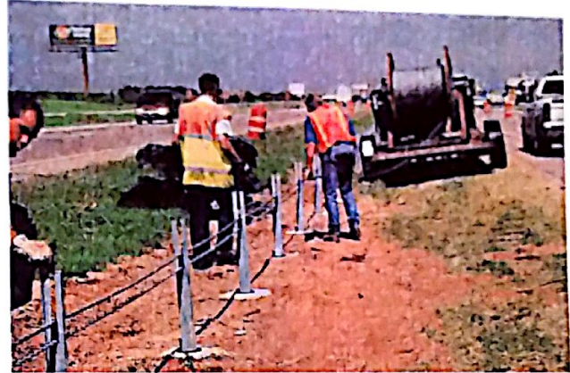
Fig. 5h: Placing second cable and inserting spacers for third cable.
