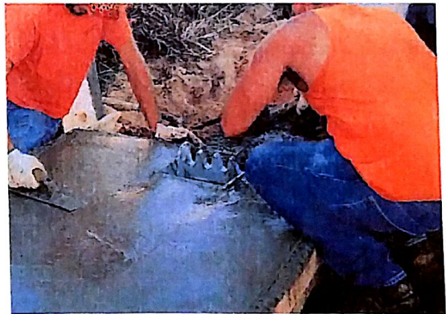
Fig. 1d: Cable anchor concrete is finished.
