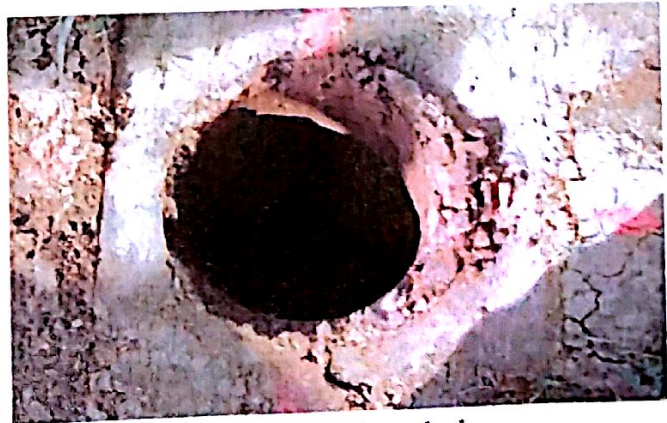
Fig. 3d: Completed post base hole.
