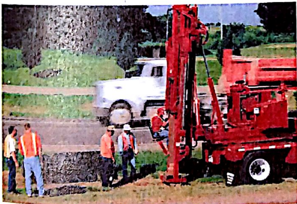
Fig. 3c: Compacting soil to form post base holes.
