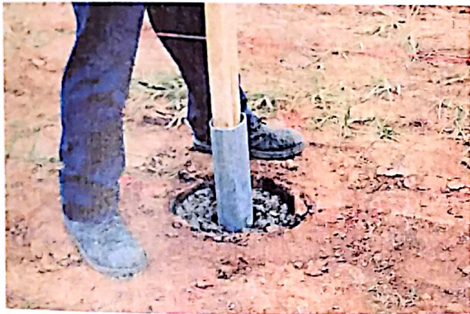
Fig. 4c: Placing post sleeve into concrete base.
