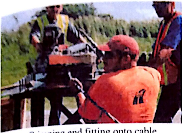
Fig. 5e: Crimping end fitting onto cable.
