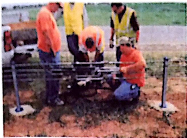
Fig. 5k: Tensioning cable three.
