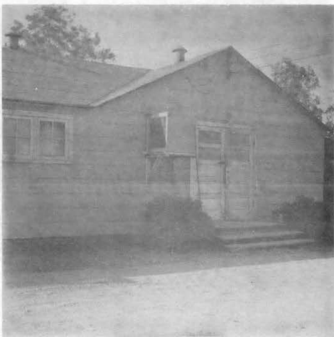
Figure 2. Building in which the Seven-Case cooler was placed.
