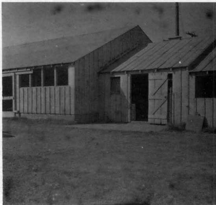
Figure 4. Location of Twenty-five case cooler.
