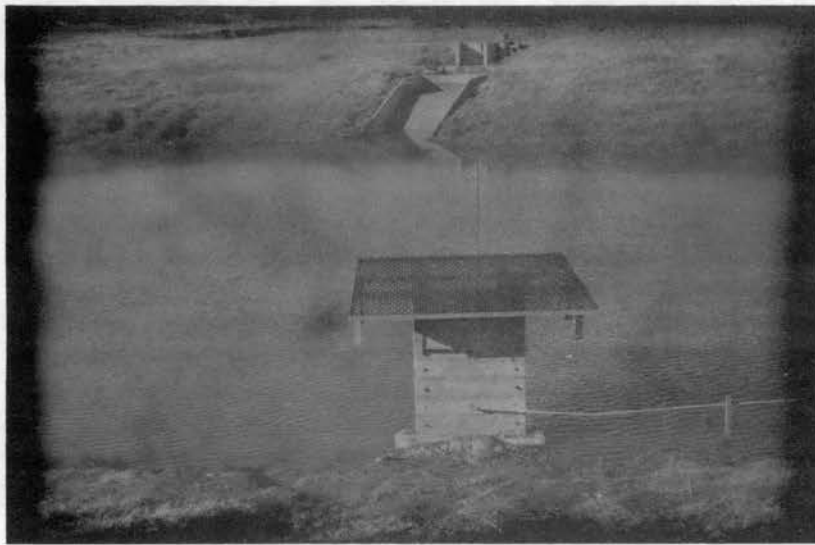
Figure 2. The steel deck grating. The water supply facilities are in the background.
