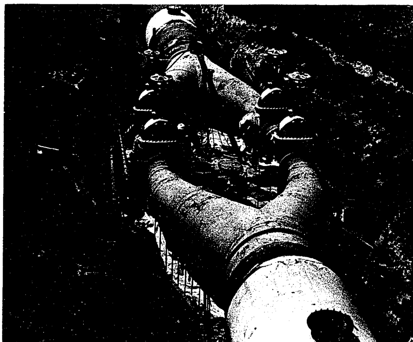
Plate 32--Amarillo turnout during construction. Wye branches and valves are in place. (Photograph courtesy of Bureau of Reclamation.)
