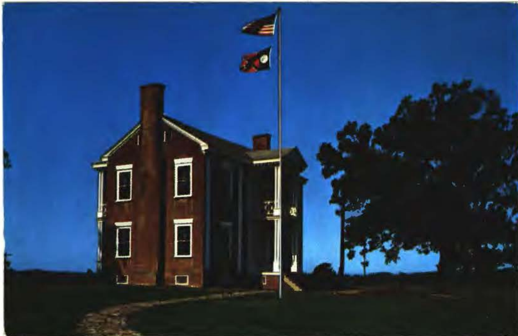
Fig. 1. North (Front) and East Elevations, Joseph Vann House, "Spring Place", Georgia
