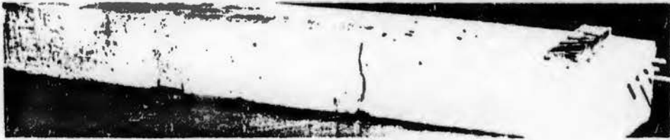
(b) Tension Failure in Concrete Underload
