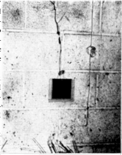
Fig. 9.—Heat flow meter installed on inside face of west wall, experimental shelter.
