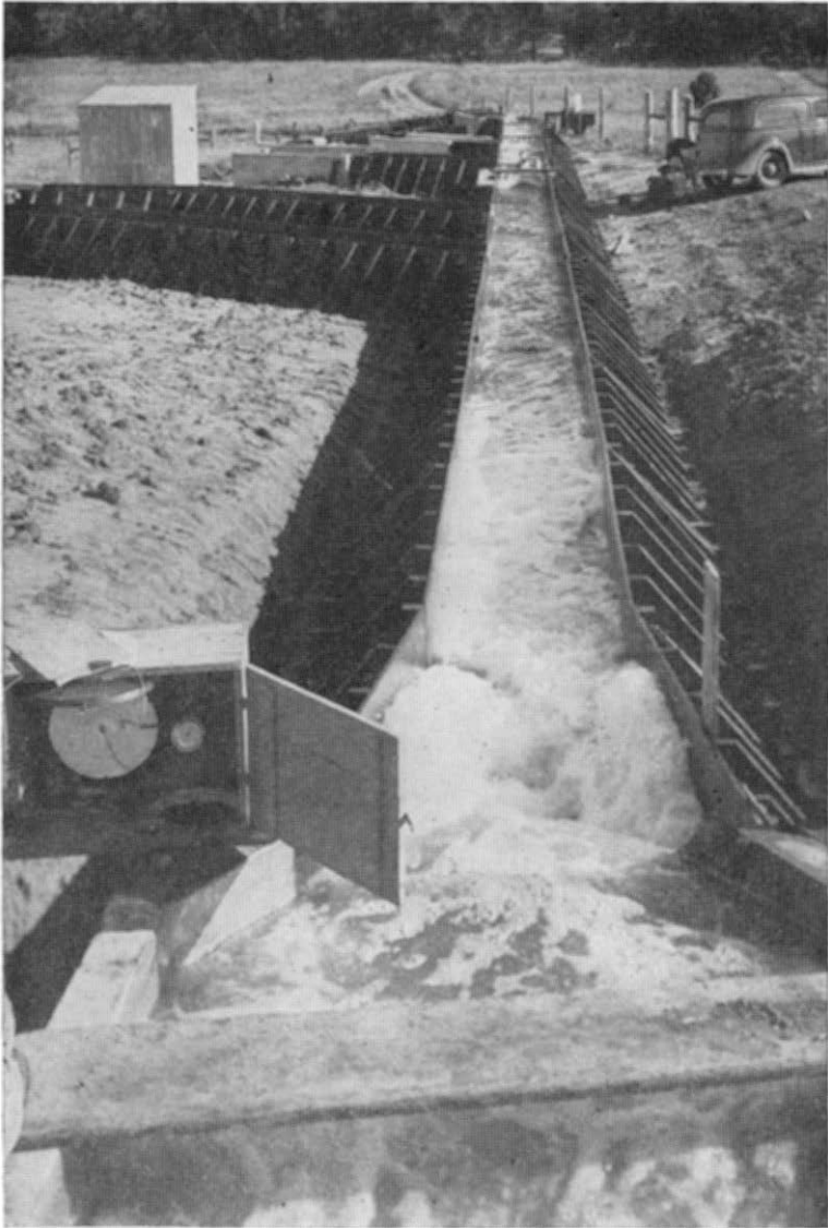
Figure 4. —A flow of 22 cubic feet per second through the type "H" rate-measuring flume and the wood flume used to convey the water to the test channels.
