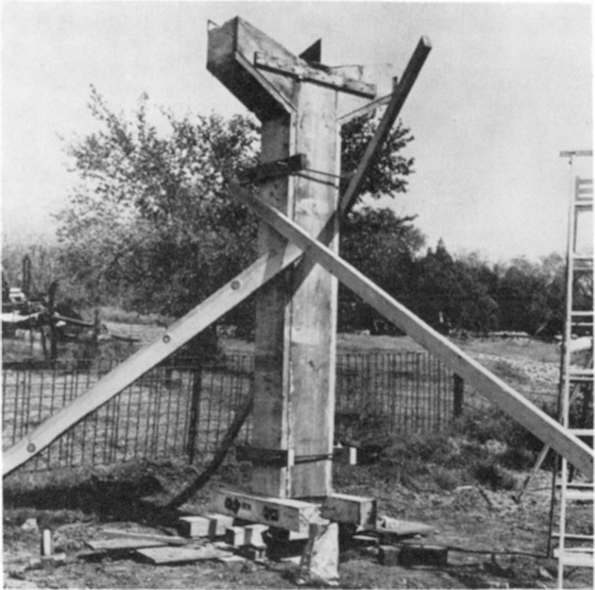
Figure 12 Precast column with temporary support.
