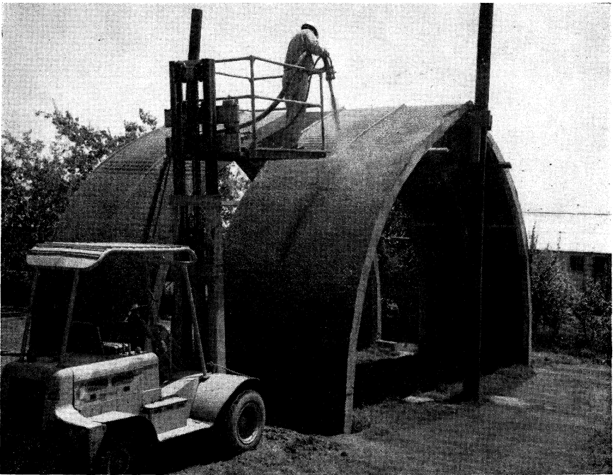
Figure 2. Pneumatic placement of wet-mix concrete for casting experimental shell arches.
