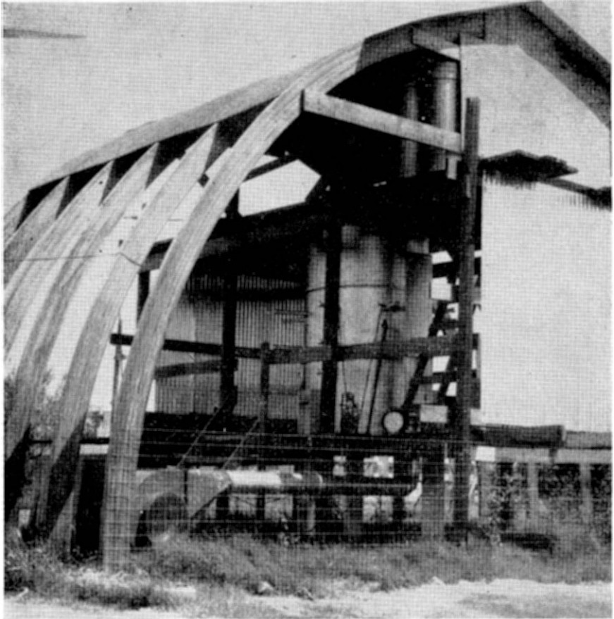
Figure 11. 4 ft. 8 in. bins installed at test site
