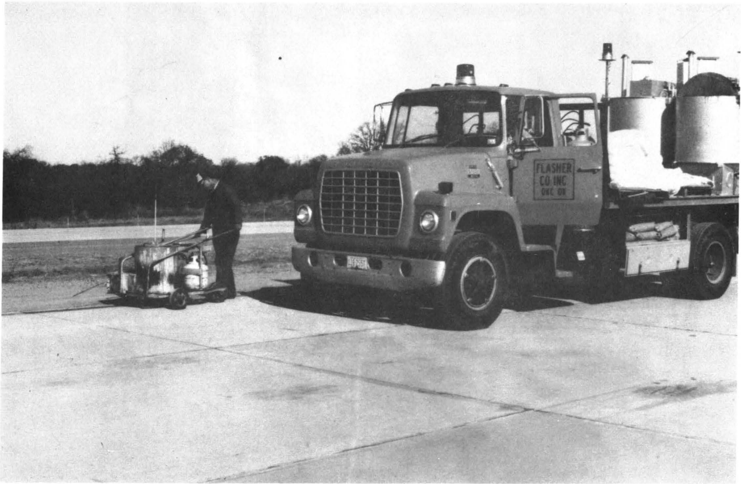
Figure 3. Thermoplastic applicator cart and furnace truck.
