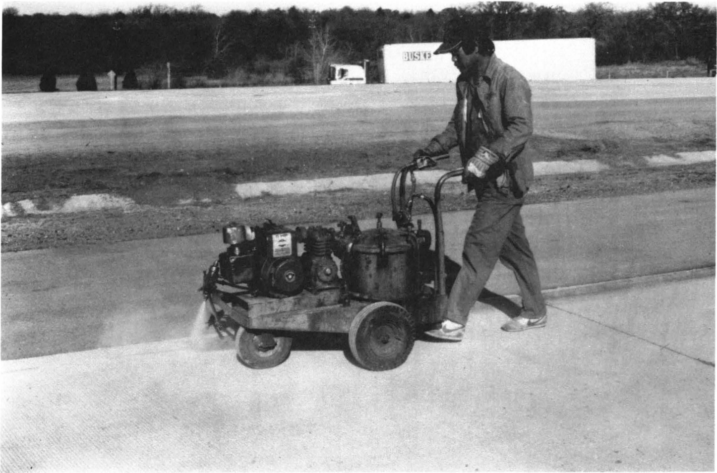
Figure 2. Applying thermoplastic primer.
