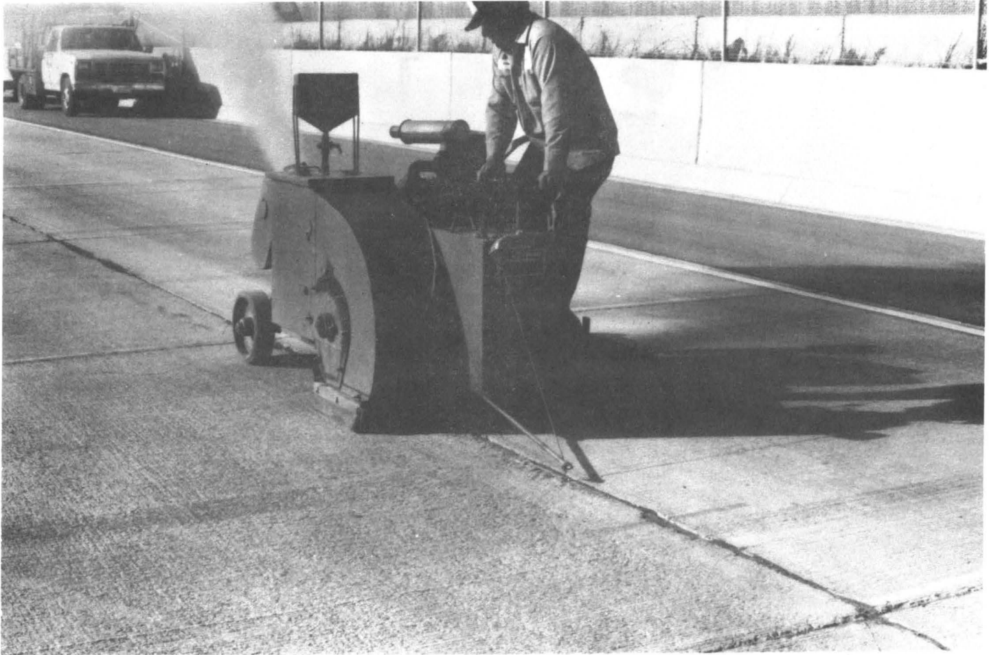
Figure 1. Shotblasting new pavement in preparation for stripe.
