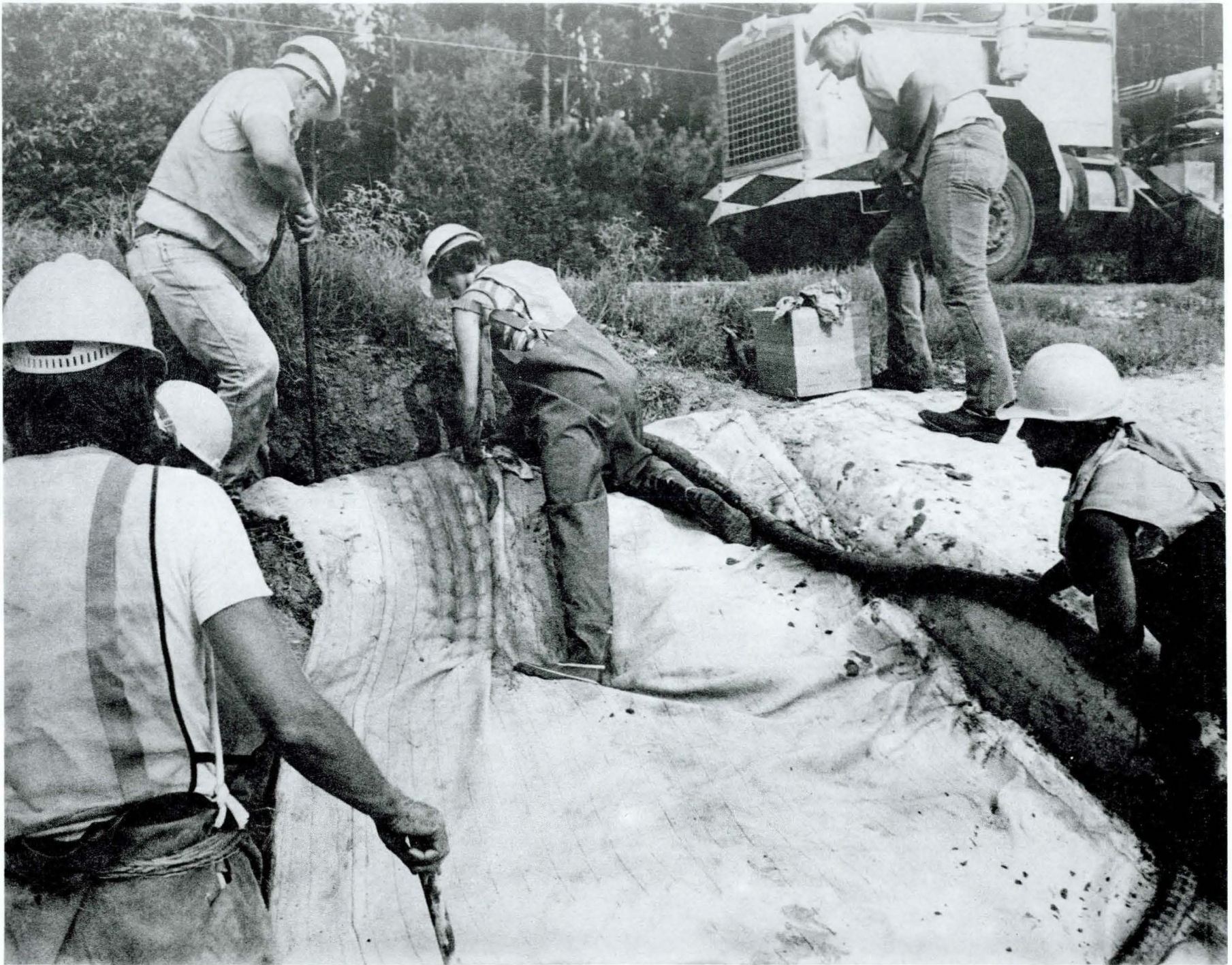
Figure 8. Filling Anchor Trenches.
