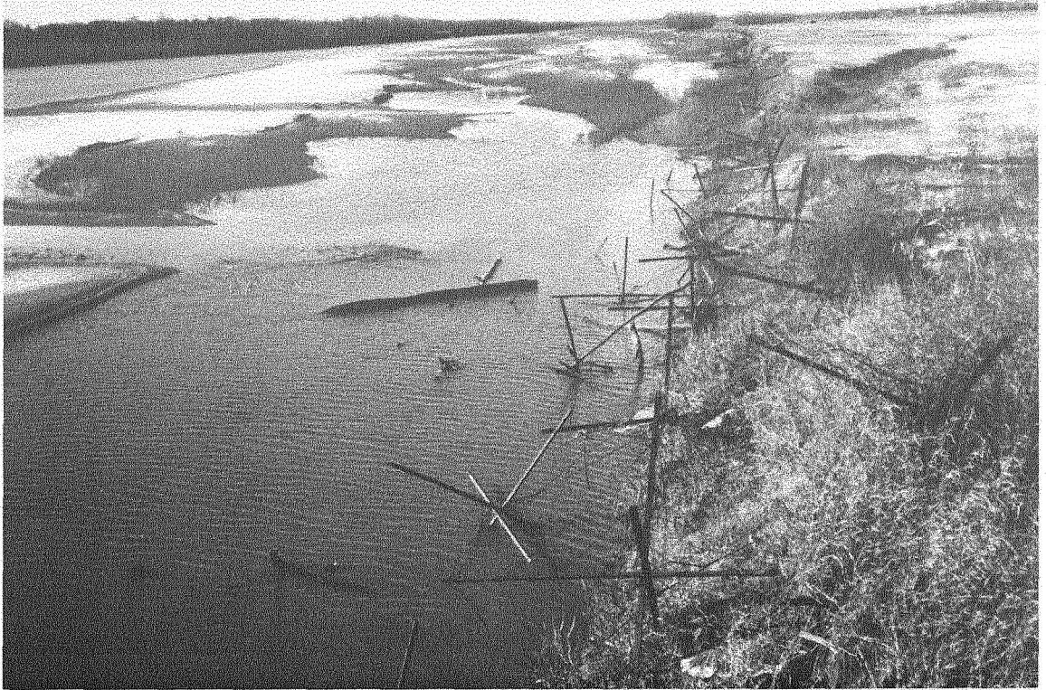
Jetty Field Upstream of Bridge
