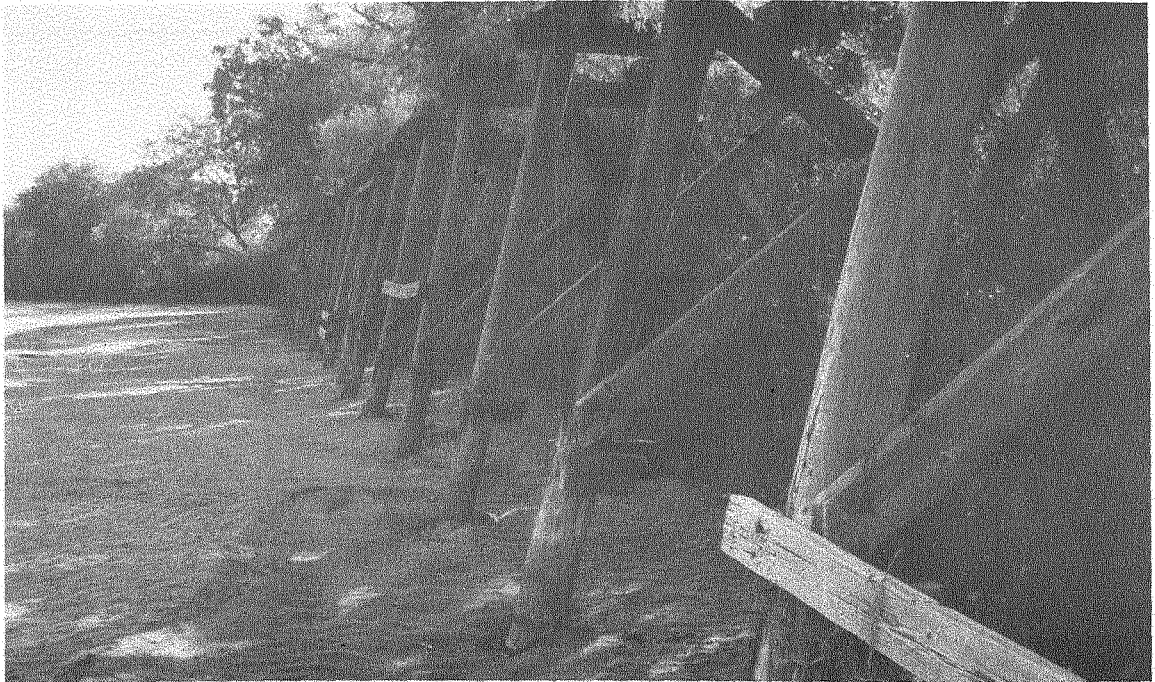
Pile Diversion with few Surface Planks
