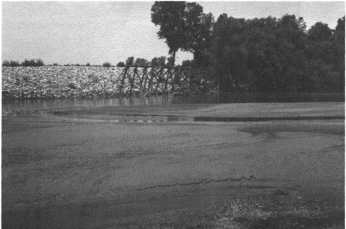
RIPRAP AND PILE DIVERSION ON WESTERN BANK
