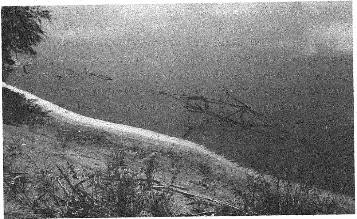
Damaged jetty fields
