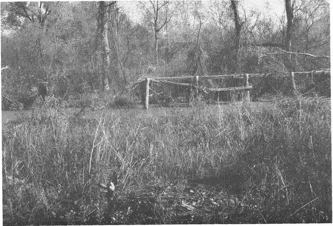
Pile Diversion standing in a Scour Pool
