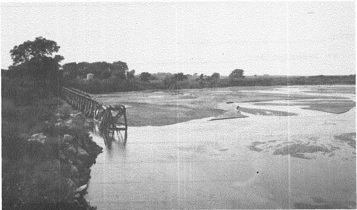
View of the Pile Diversion Field
