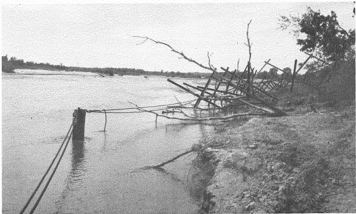
View of Mainline Jetty With Pile Anchor
