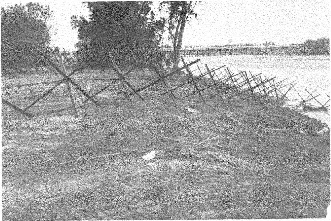
View of Bridge from Jetty Field
