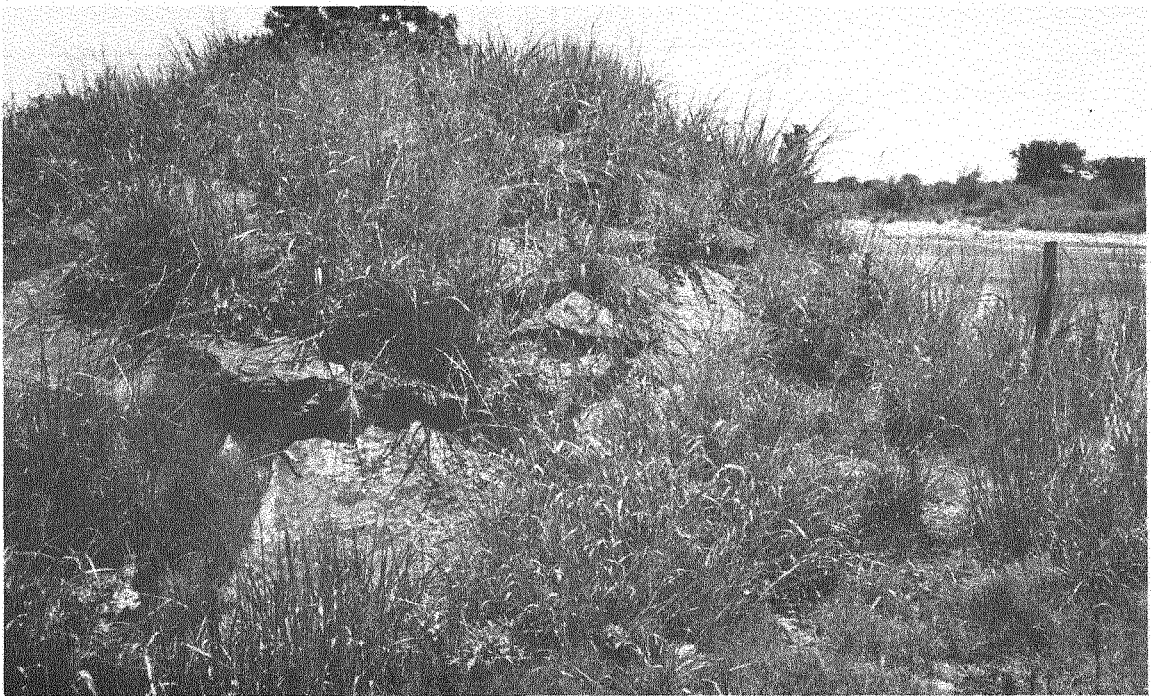
Dike with a Facing of Riprap
