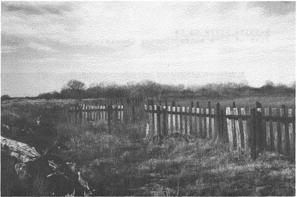
Henson Type Fence Structure
