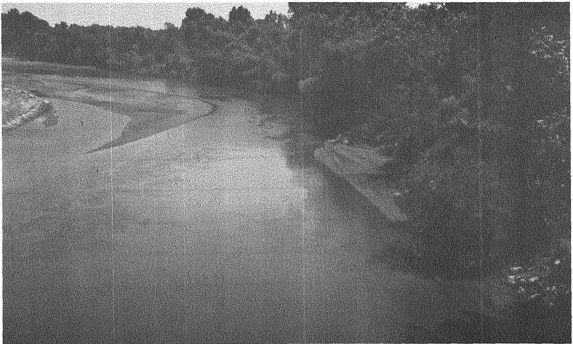
RIVER FLOW AGAINST THE EASTERN EMBANKMENT
