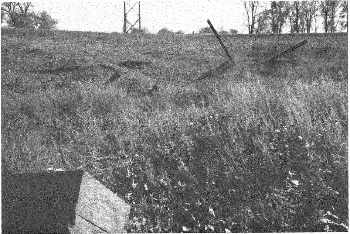
Damaged Jetty Field
