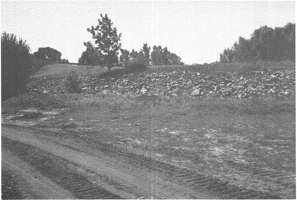
Riprap on Abutment
