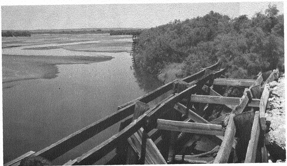
Bank Building Process in between Pile Diversions
