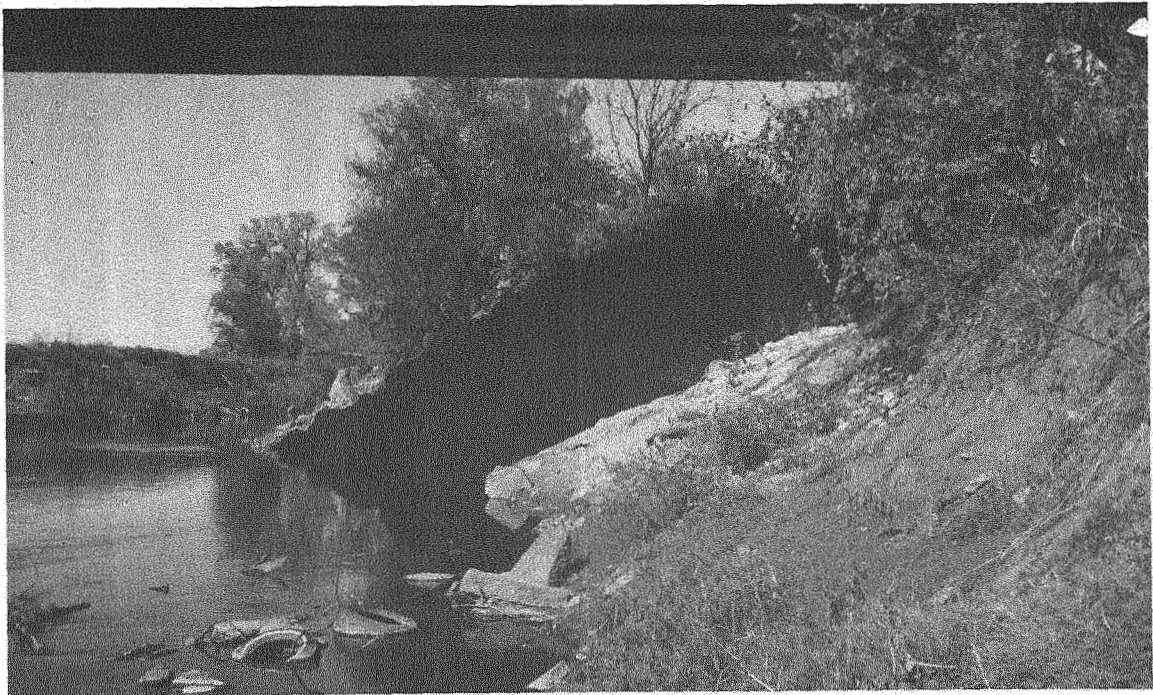
Remnants of Old Bridge
