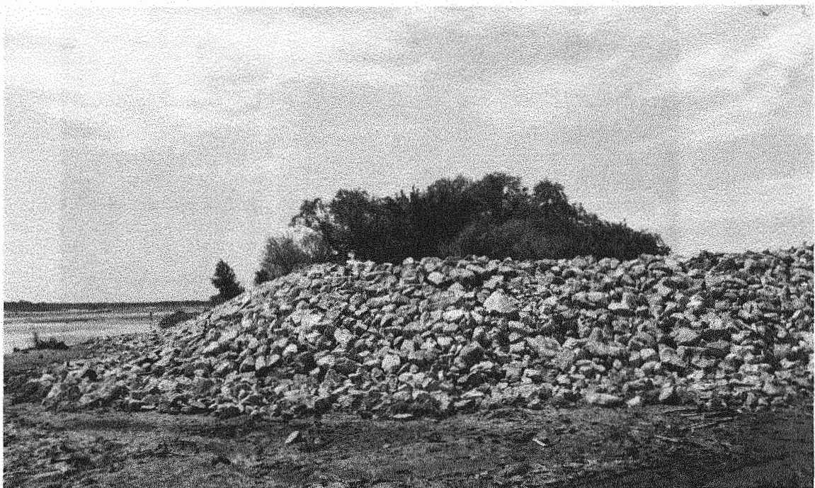
Riprap at Upstream End of Jetty Field
