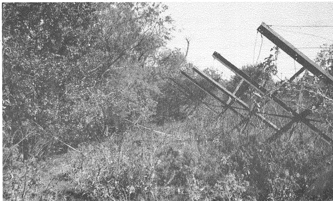
View of Kellner Jetty Field
