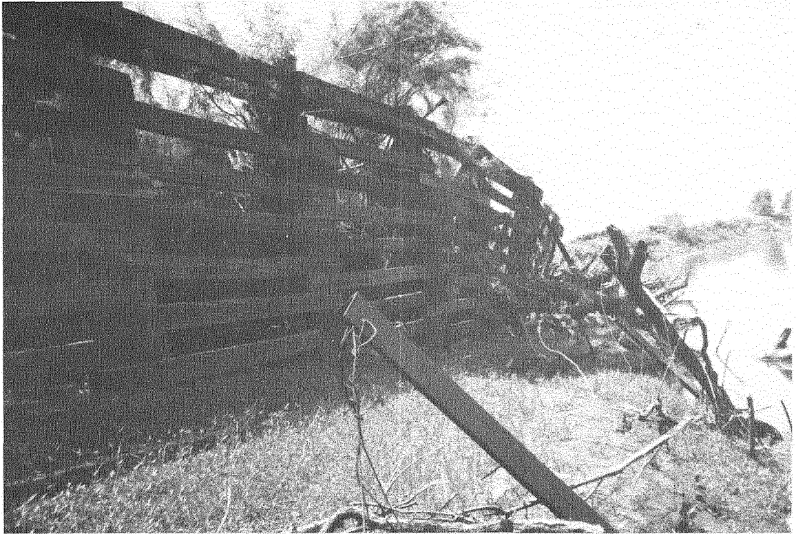
Closeup of Pile Diversion
