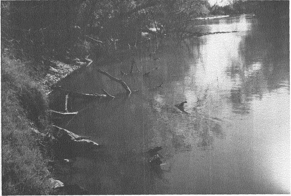
Damaged Kellner Jetty Field
