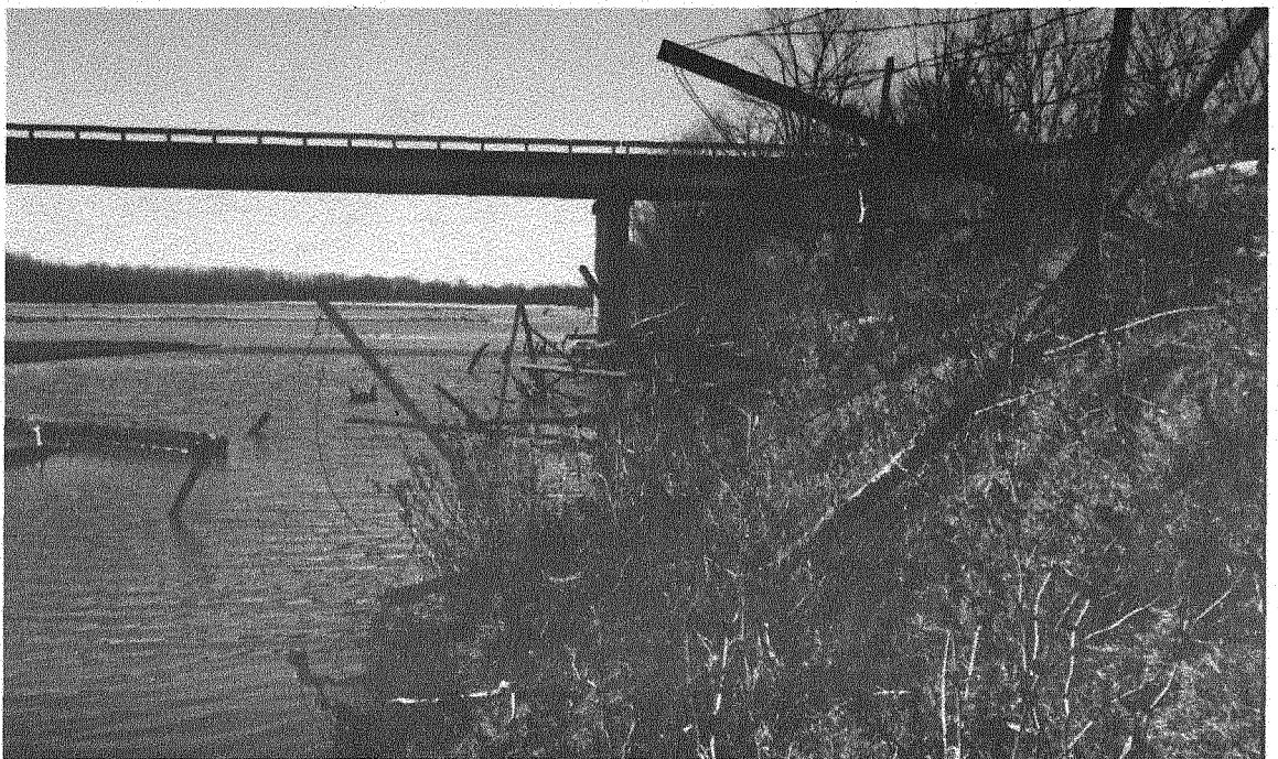
Jetty Field Downstream Of Bridge
