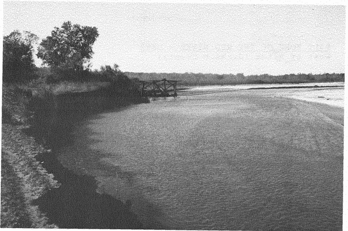
View of Eroding South Bank (Upstream)
