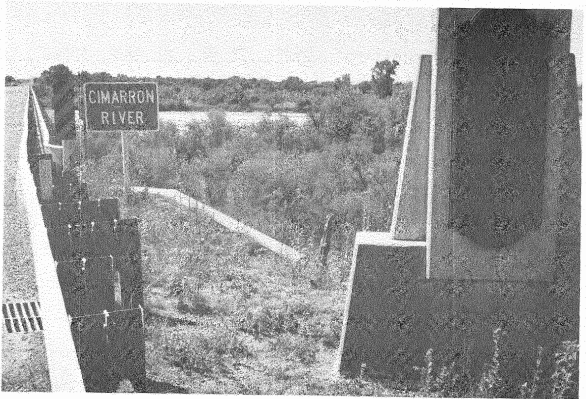
View of Bridge Site
