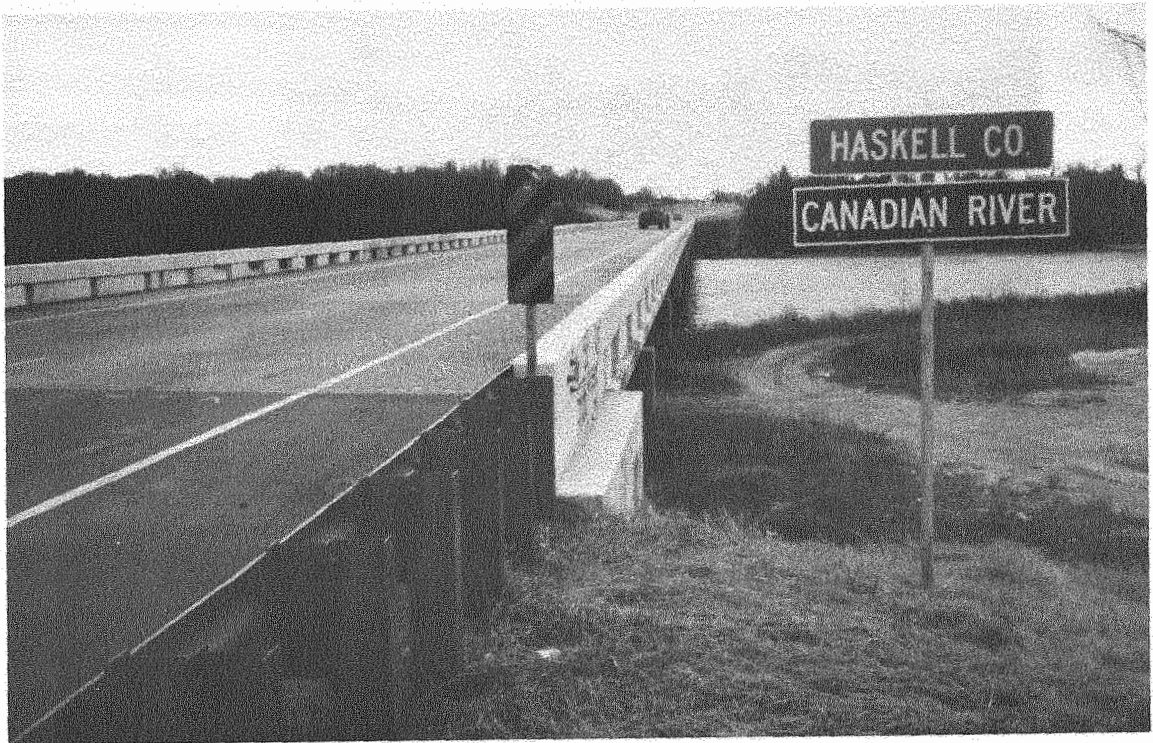
View of the Bridge Site
