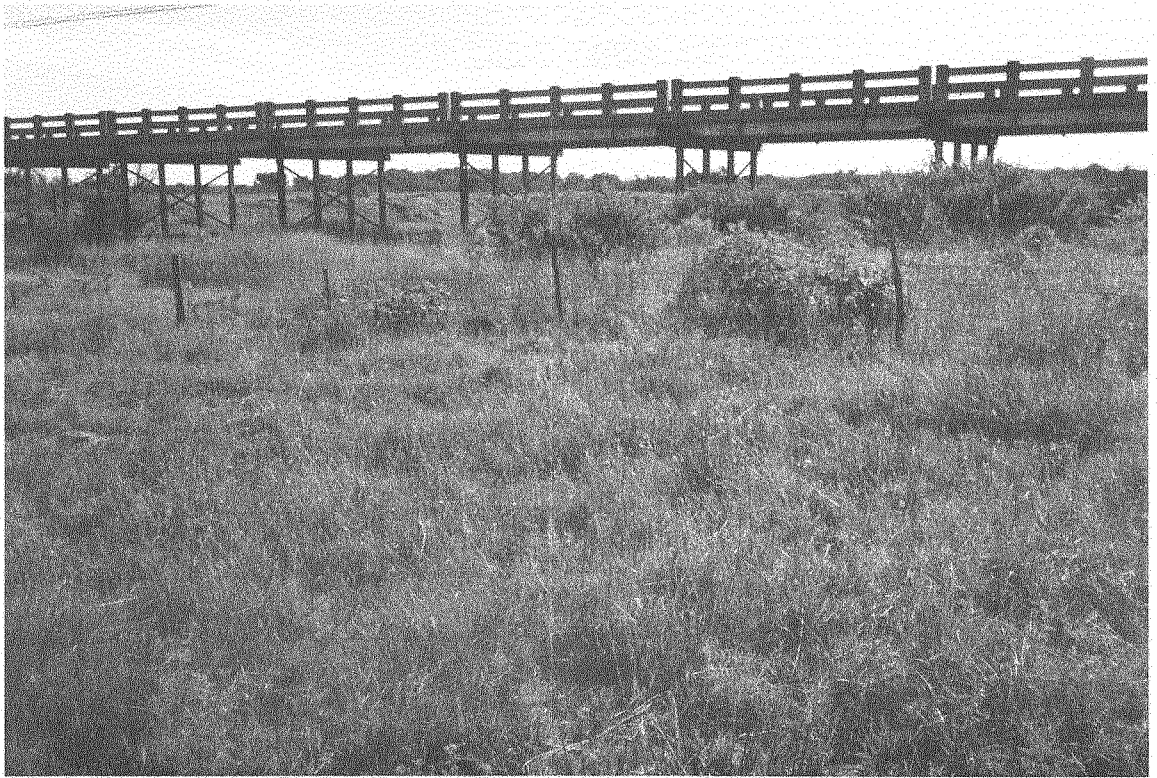
View of Bridge Site
