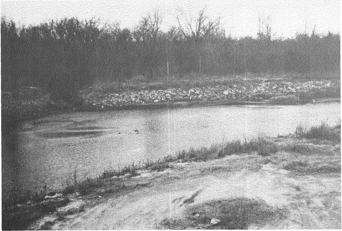
Riprap on the Upstream Bank
