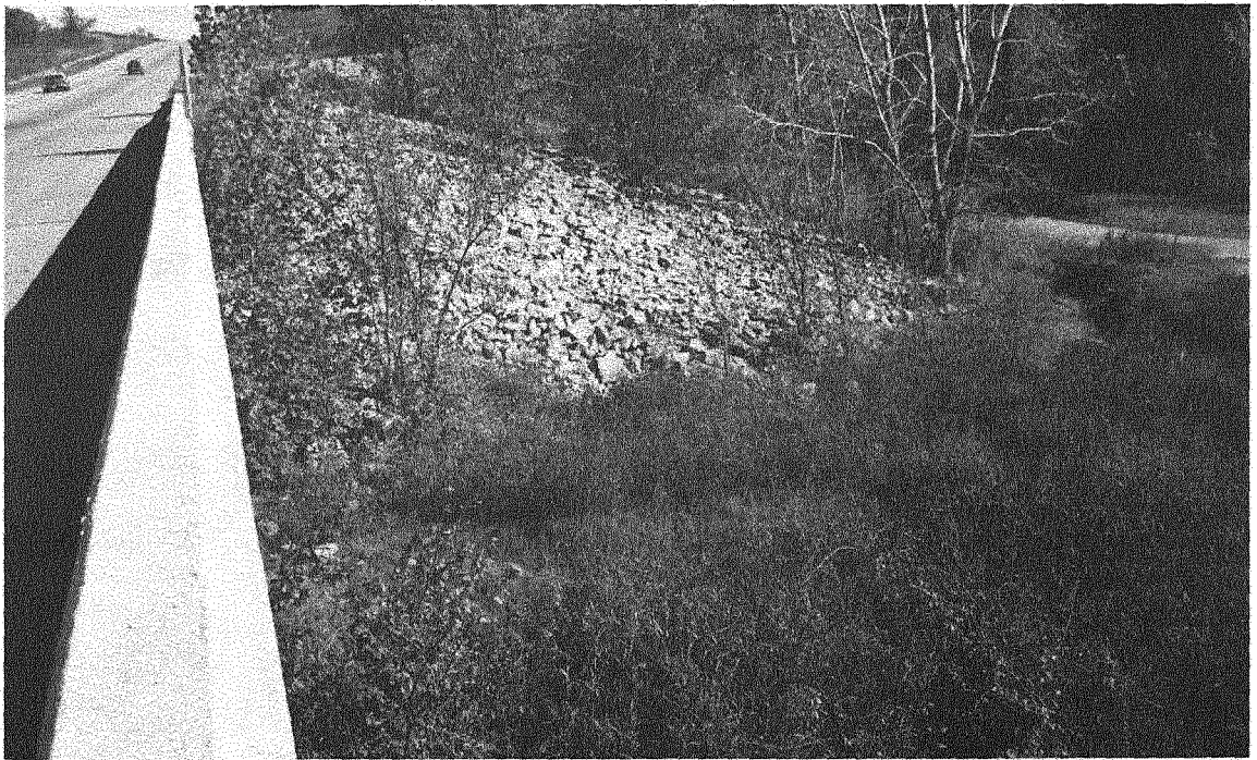
Riprap At Bridge Abutment
