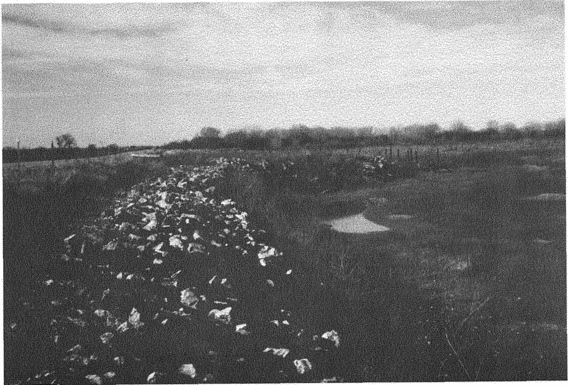
Massive Riprap Along the Highway
