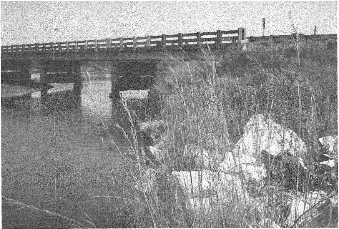
View of Bridge Abutment with Riprap
