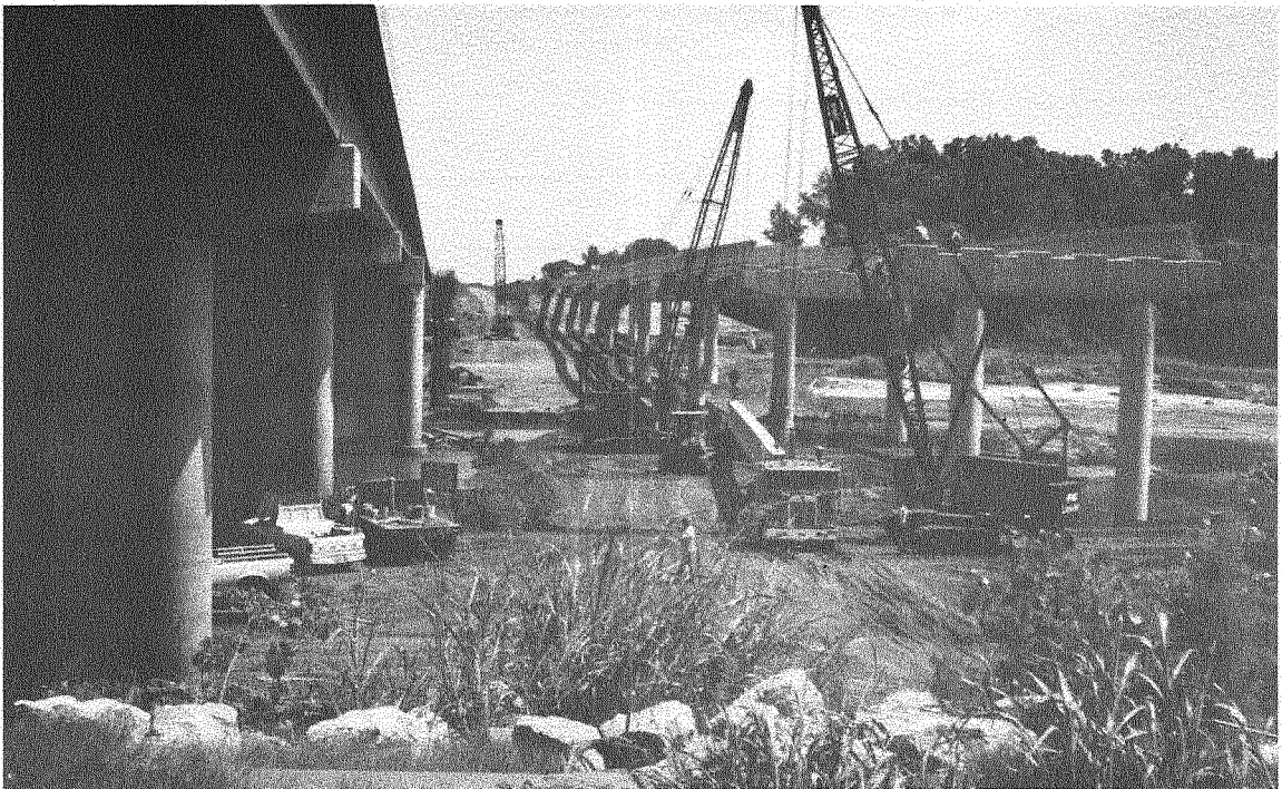
New Bridge Under Construction
