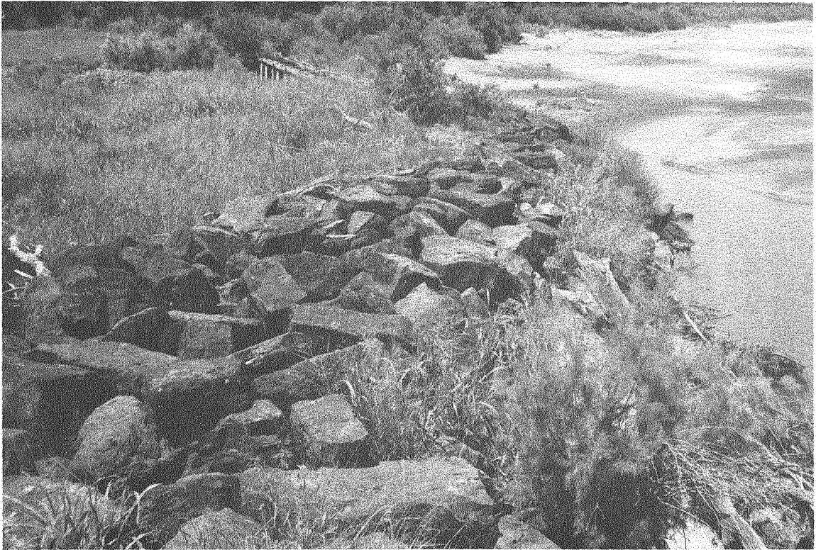
Riprap on the Southern Abutment
