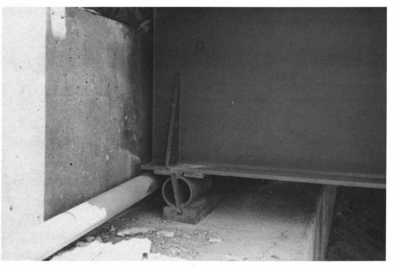
Fig. 3. An expansion device showing extensive tilting.
