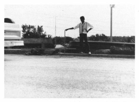
Fig. 4. Settlement estimate of bridge approach from the differential settlement of the curb.
