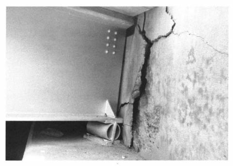
Fig. 2. An abutment headwall showing extensive cracking.
