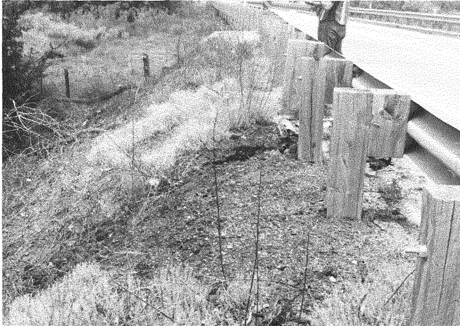
Fig. 2-2. Approach guardrail used during the period 1960-1980
