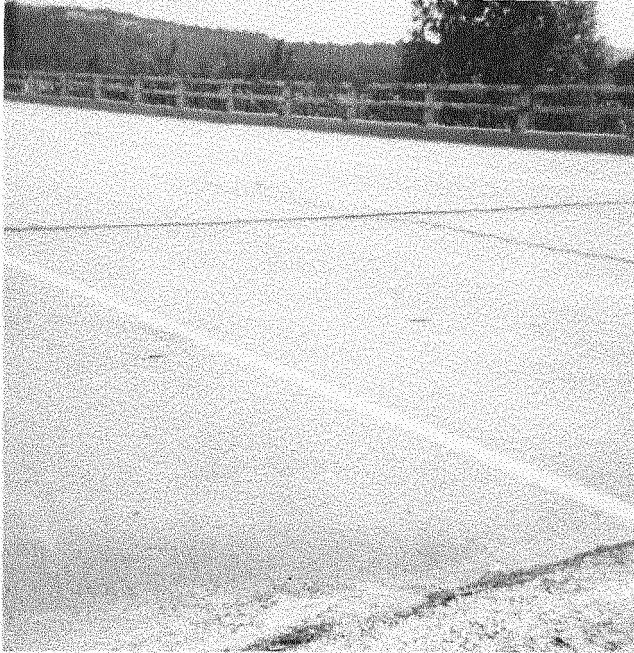
Fig. 2-6. A smooth bridge approach
