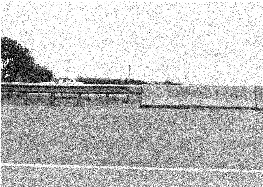
Fig. 2-3. Approach guardrail used since 1980
