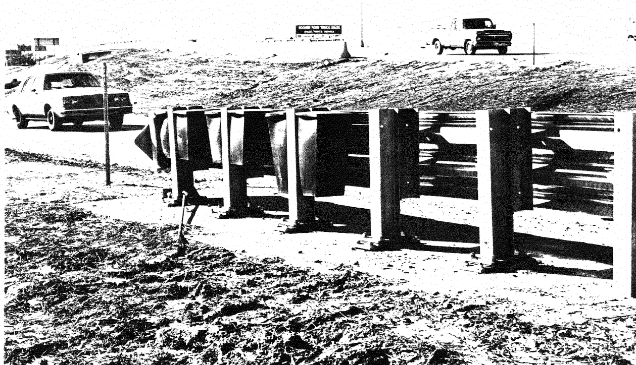
Figure 1. SENTRE unit after installation on guardrail end.
