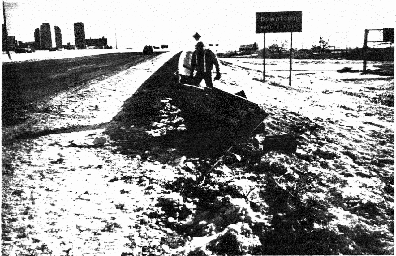
Figure 7. After collision - unit functioned as intended.
