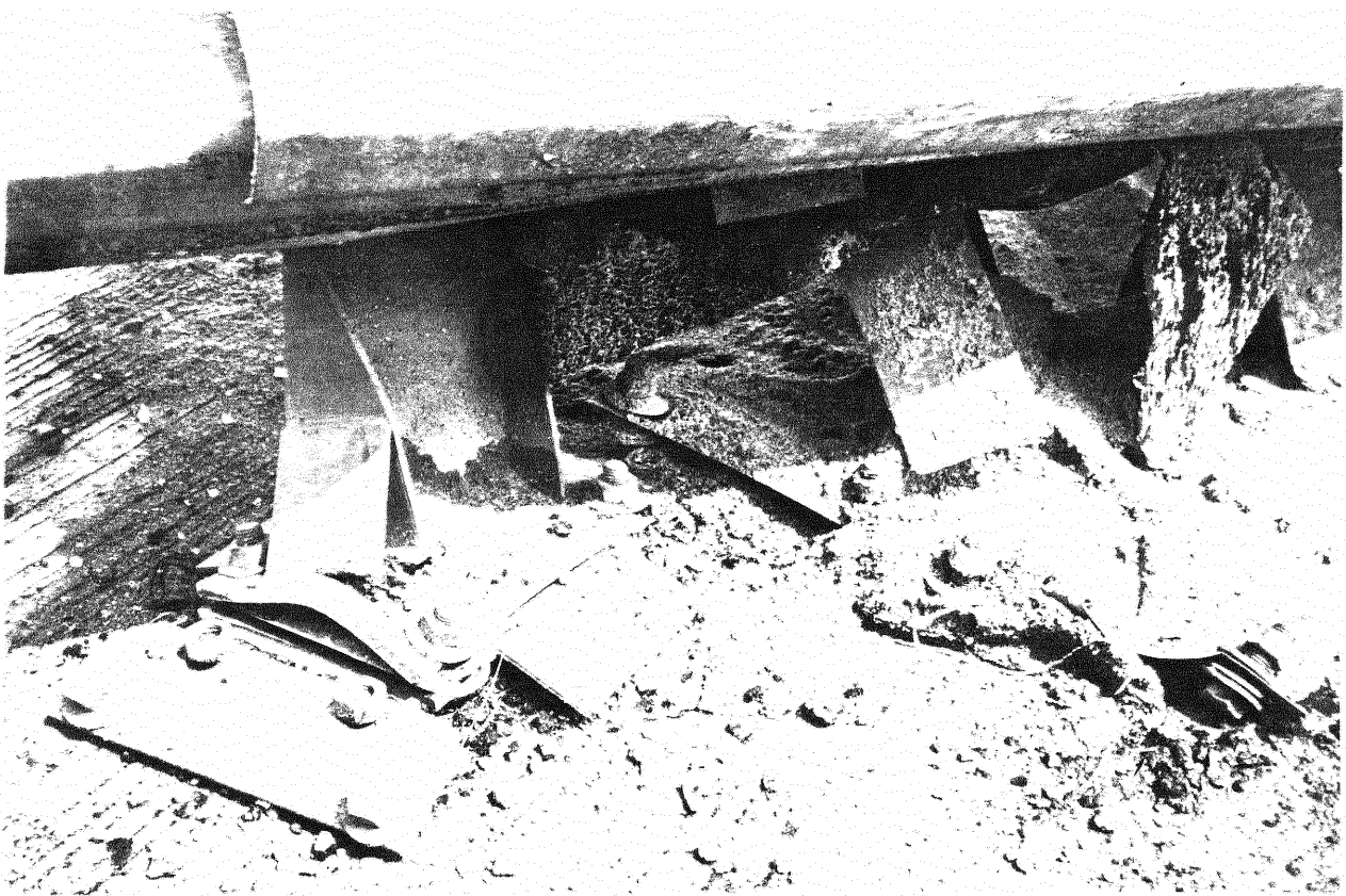
Figure 11. Slip base after impact, base did not perform.
