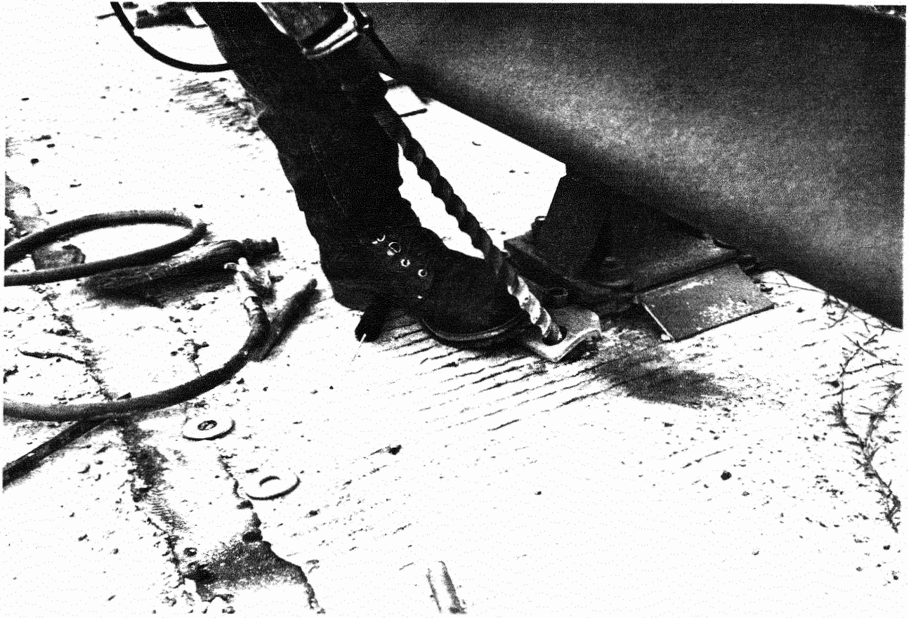
Figure 3. Drilling holes for "MP-3" anchors during retrofit.
