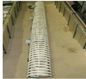
(b) Spiral-coil type GHE setting
