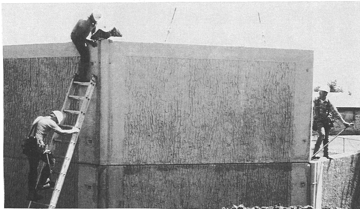
Figure 15. Guiding FANWALL Panels into Place.
