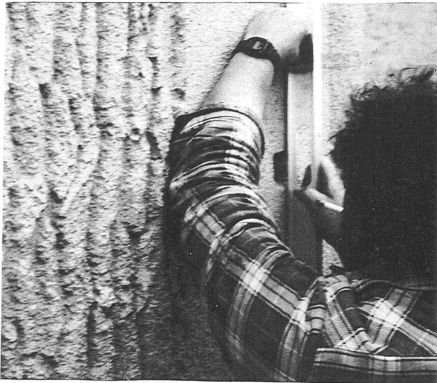
Figure 23. Making Measurements Used to Monitor FANWALL for Tilting.
