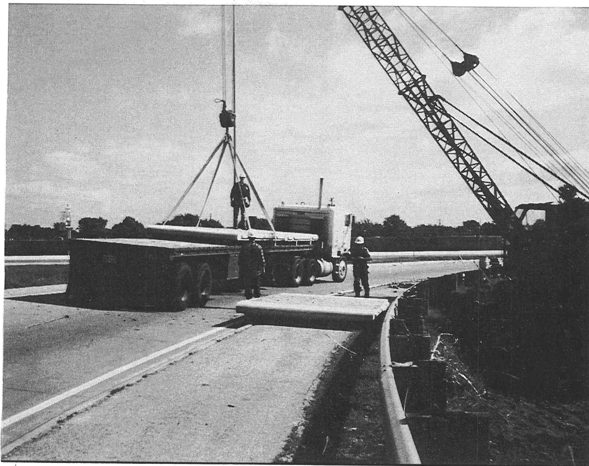
Figure 10. Unloading FANWALL Panel with Lifting Straps.
