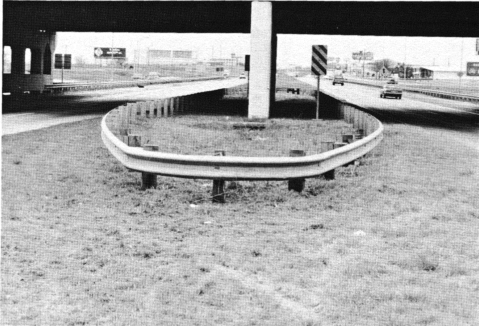
FIGURE 2.8 Parabolic end
