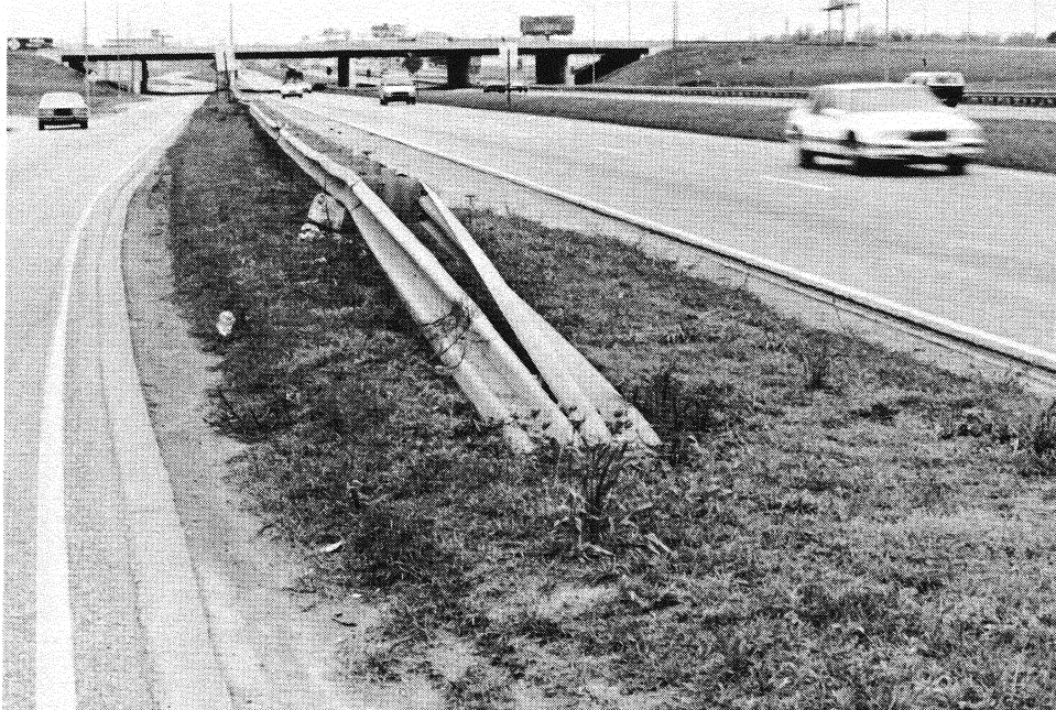
FIGURE 2.5 Double-faced turned-down end treatment
