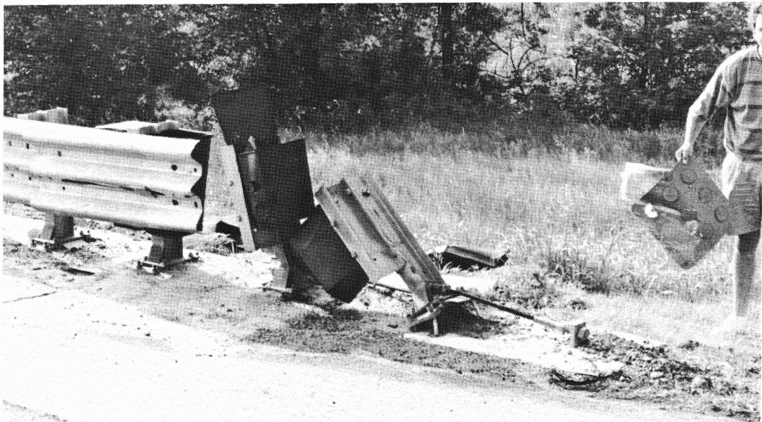
FIGURE 2.7 Sentre impact on Oklahoma turnpike
