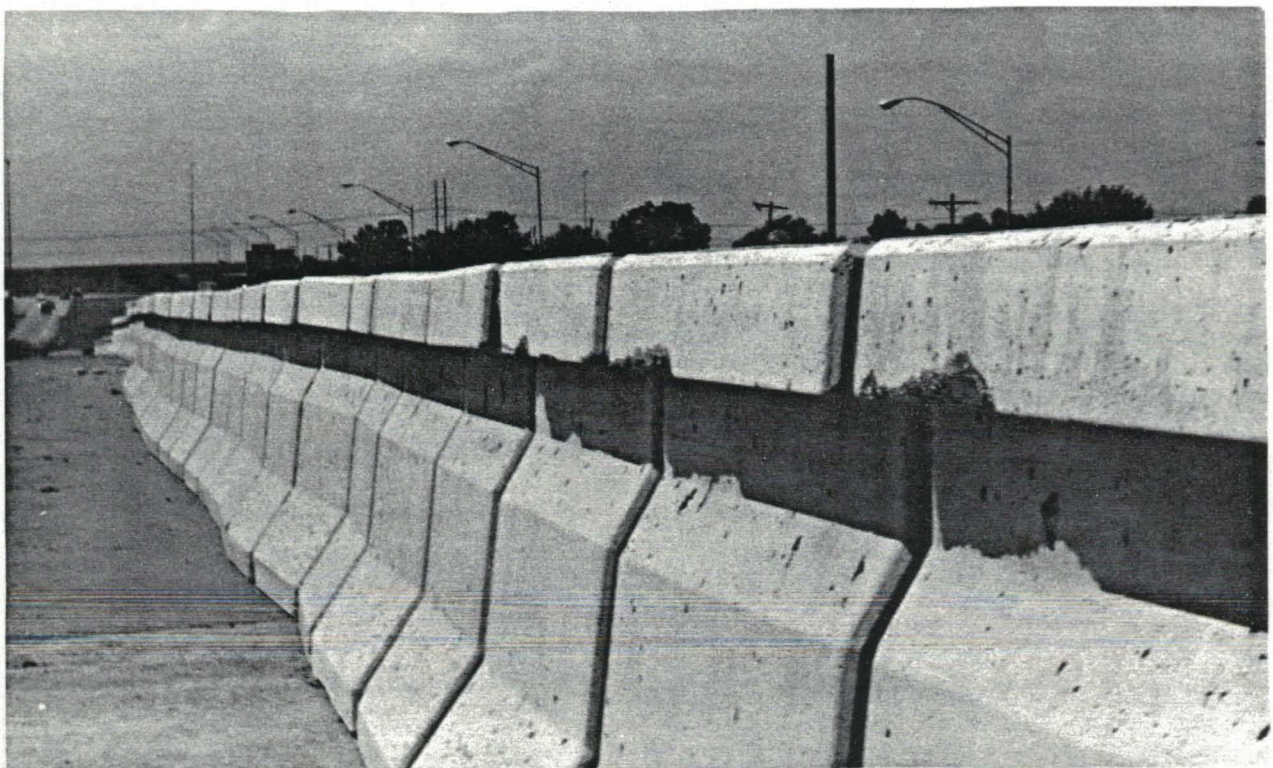
Figure 13. Chipping Under Flanges on Barrier Segments.
