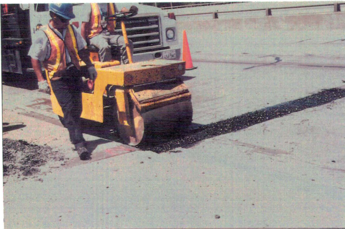
Figure 13. Compacting Modified AC with Two Ton Roller
