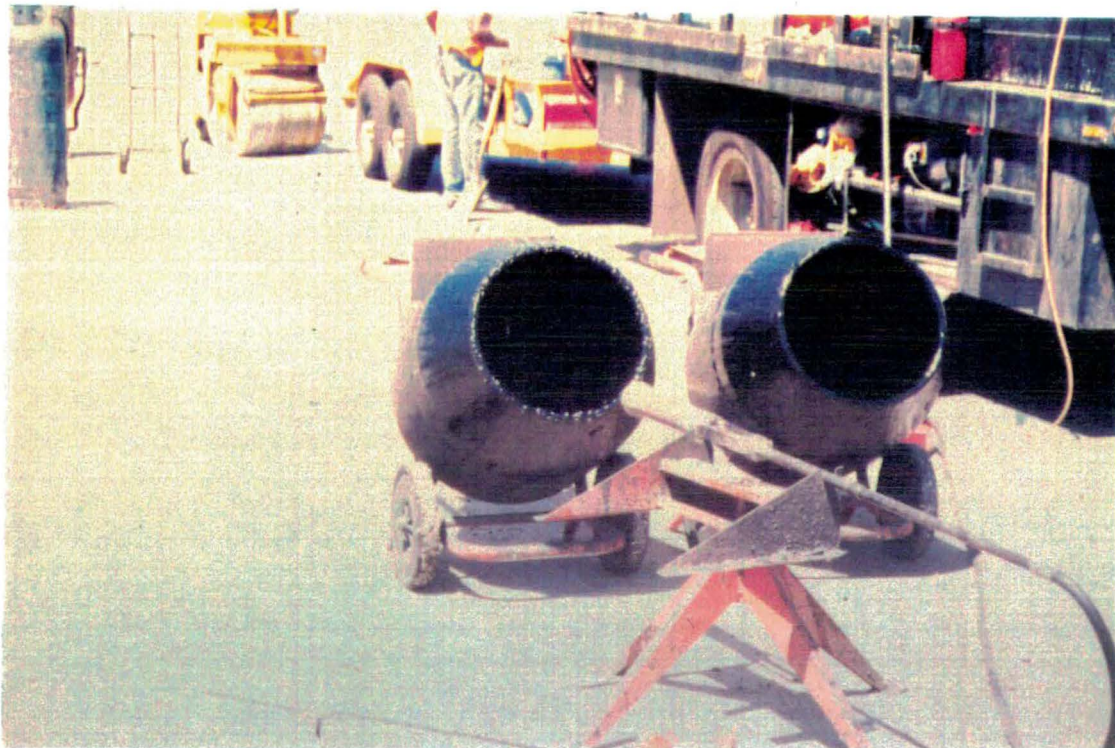
Figure 10. Mixing BJB and Granite Aggregate in 1/2 C.Y. Mixers.
