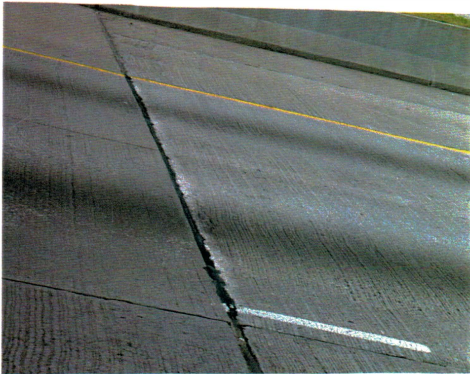
Figure 19. Expansion Joint Sealed with Self-Levelling Sealant.
