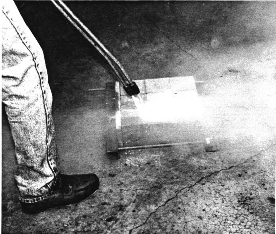
Fig. 3.11 High Pressure Water Washing, Phase III Cubes
