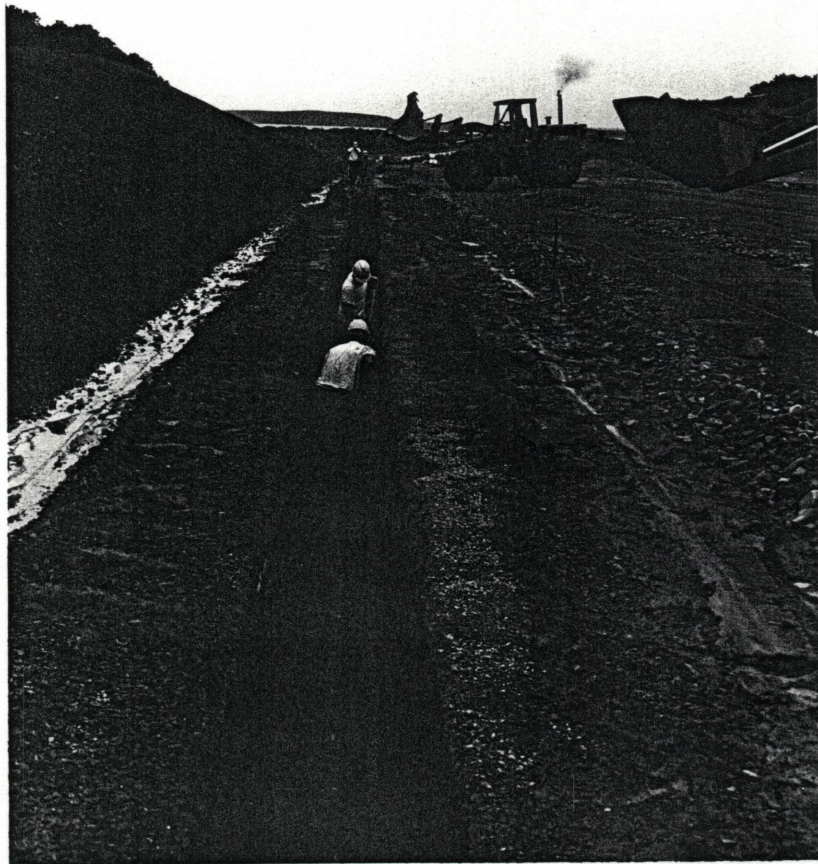
The pipe is covered with a second layer of bedding material.
