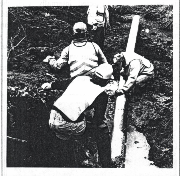
Figure 29 Installing CGMP outlet.
