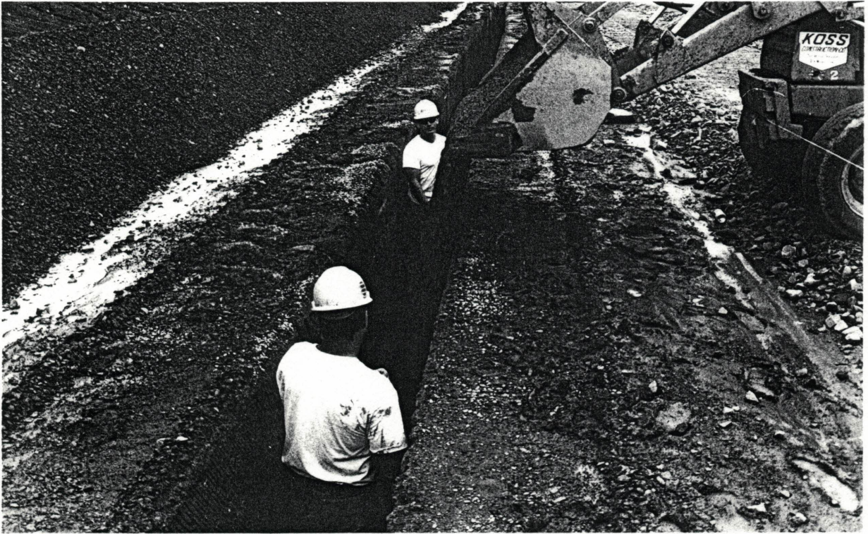
The bottom of the trench is layered with bedding material.
