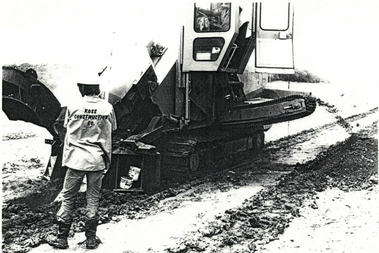
The spoils are ejected via conveyor belt.
