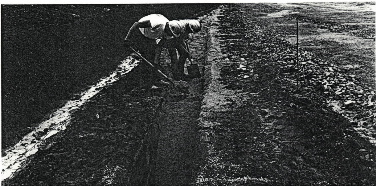
Filter sand comes to within 15 cm of the top before the trench is capped with spoils.
