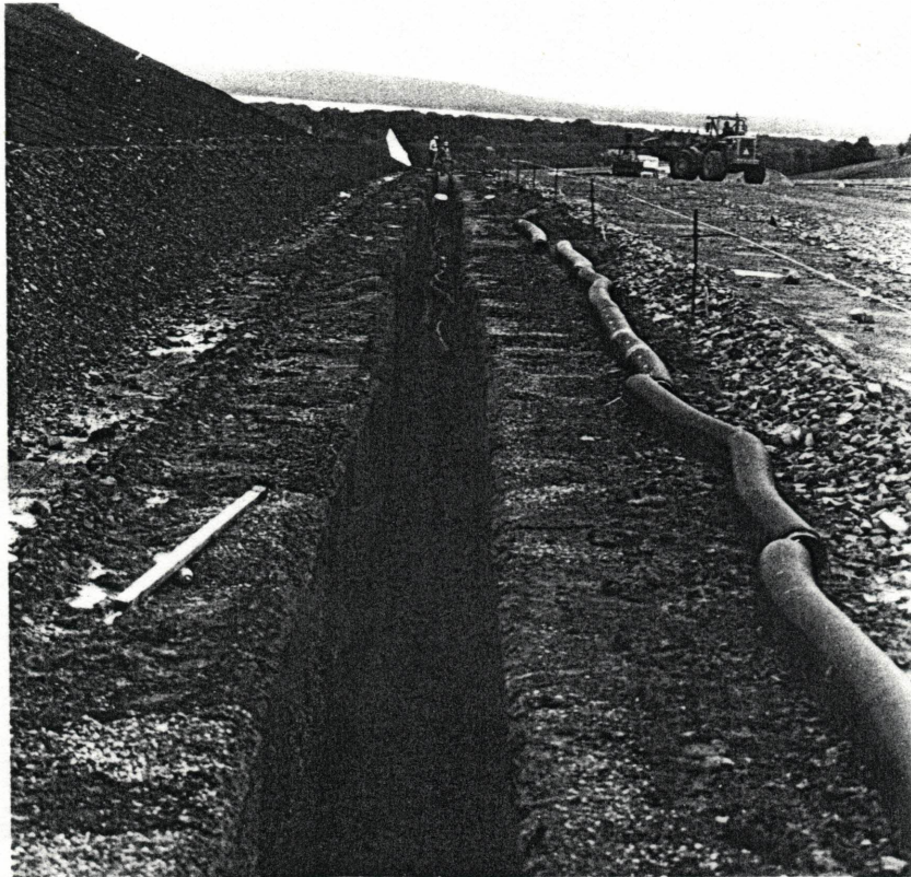
The perforated underdrain pipe is laid in.
