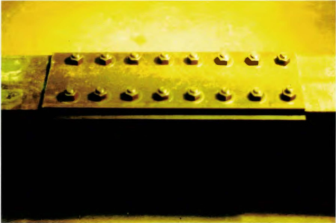
Figure 71. Splice Plate Detail
