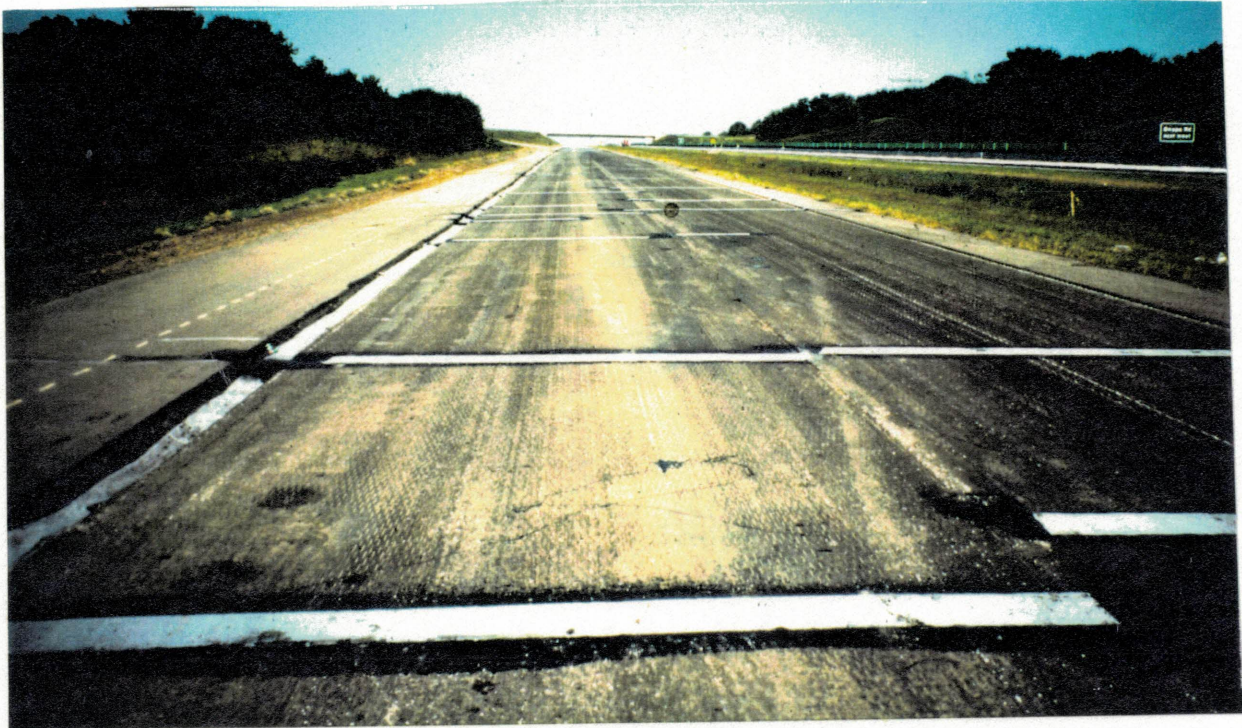
Figure 14. Pro-Guard After Application.
