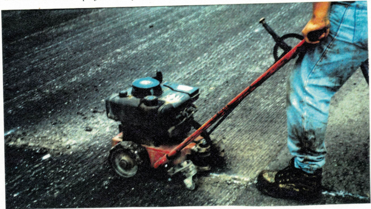
Figure 9. Routing Cracks.
