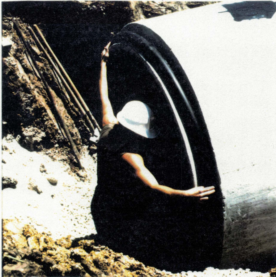
Figure 1. Placing Omni-Flex Seal on RCP section.
