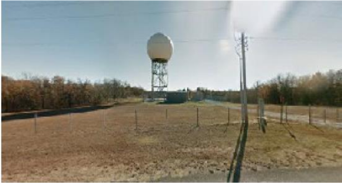
Fig. 3. 1 Street View of KTLX WSR-88D radar
