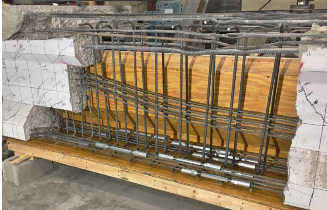
Figure 5.32 North End Girder Internal Reinforcing
