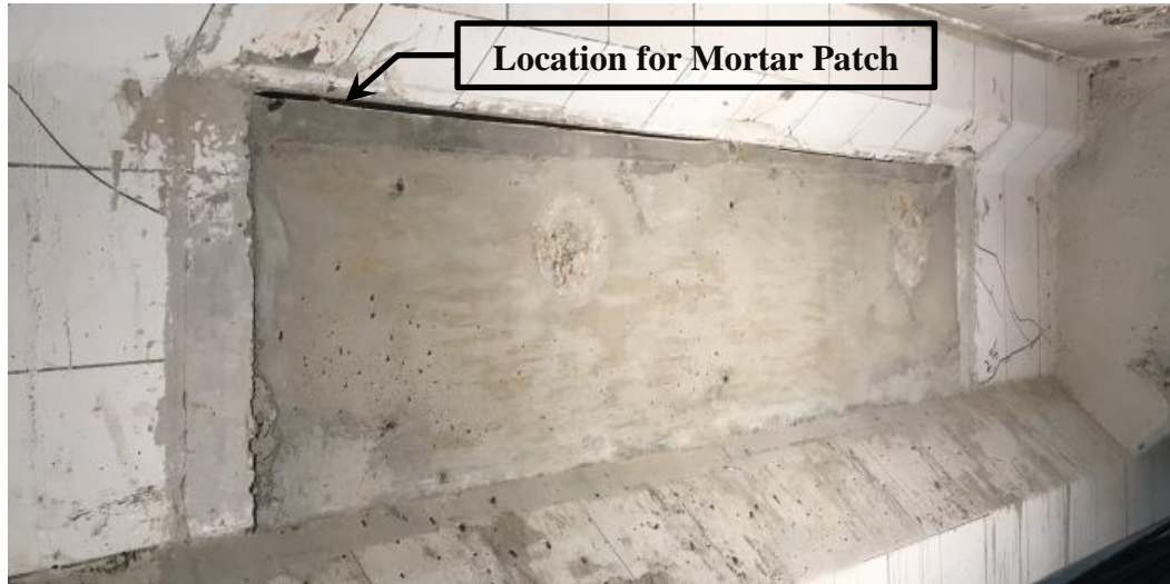
Figure 5.6 Core-Sampled Finished Repair (Without Mortar Patch)
