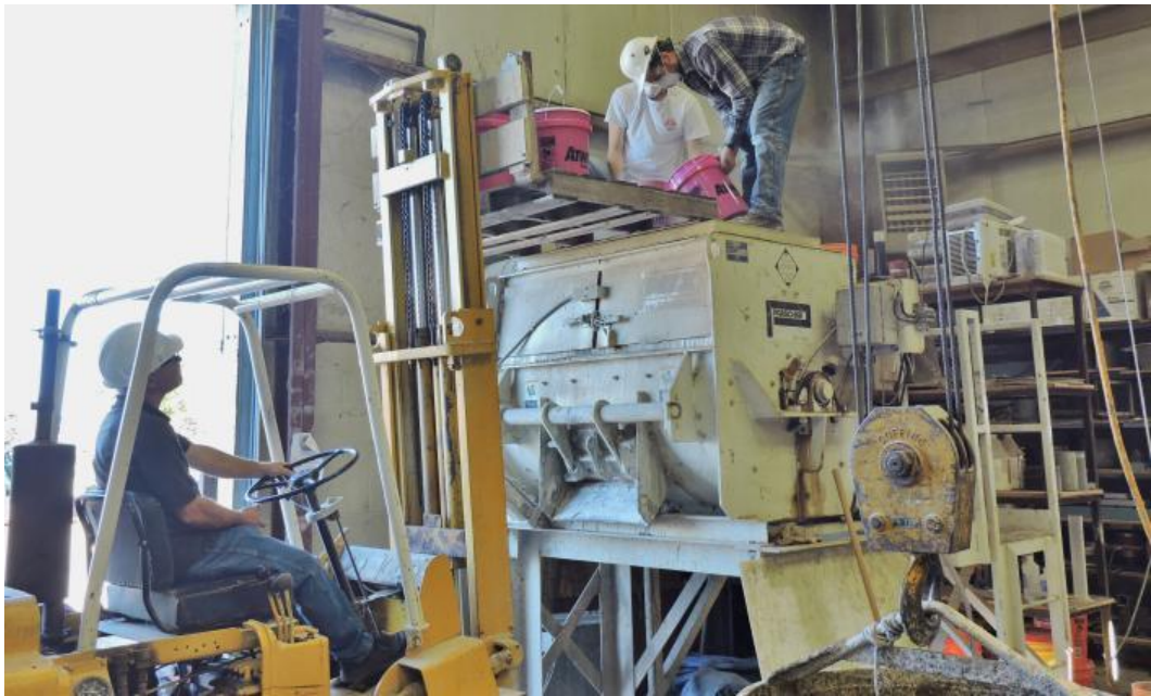
Figure D.2 Adding Cementitious Material During the Mixing Process
