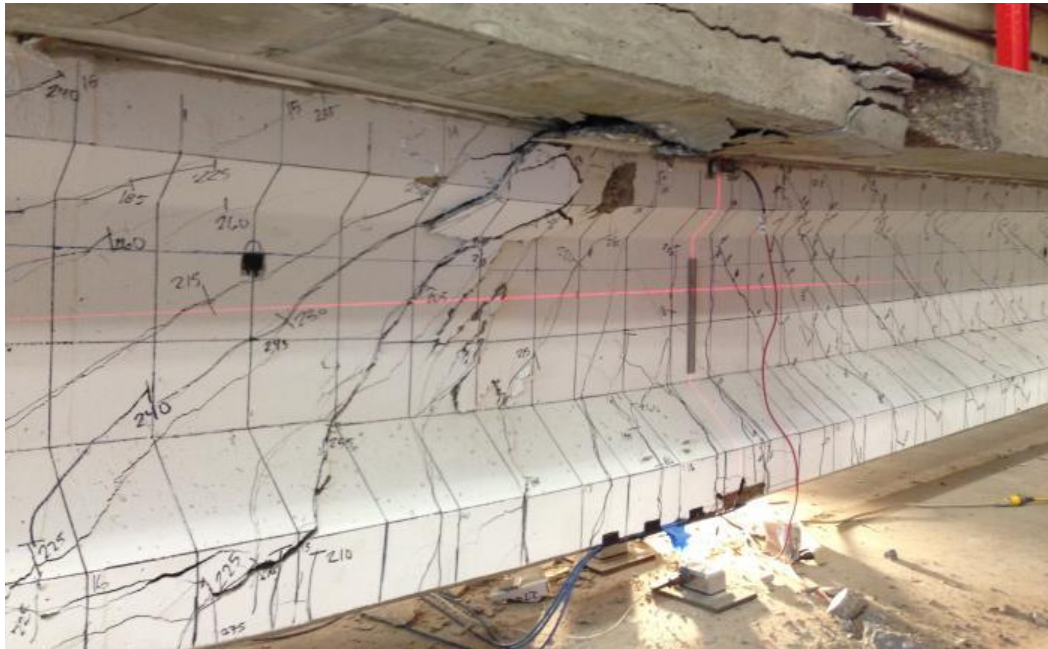
Figure 4.8 Cracking During Test C2
