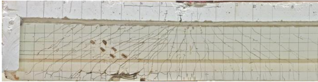
Figure 5.7 South End Damage From Original Testing
