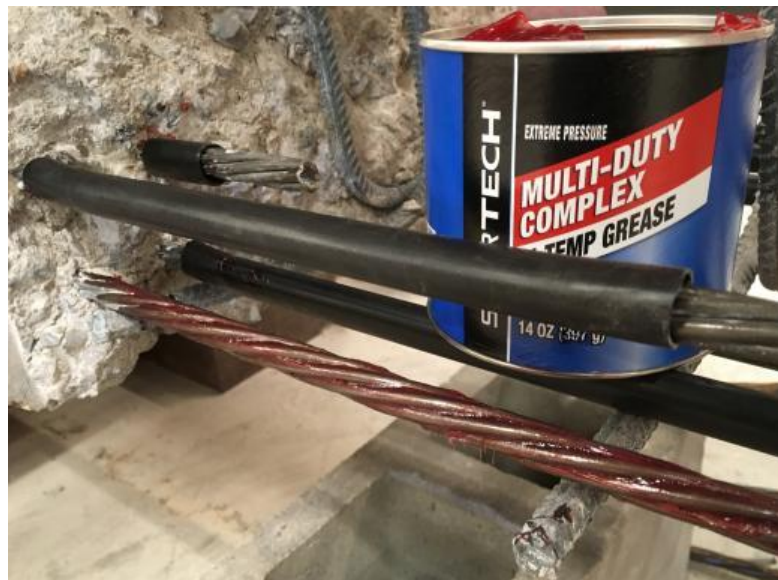
Figure 5.12 Post-Tensioning, Grease-and-Sleeve Arrangement
