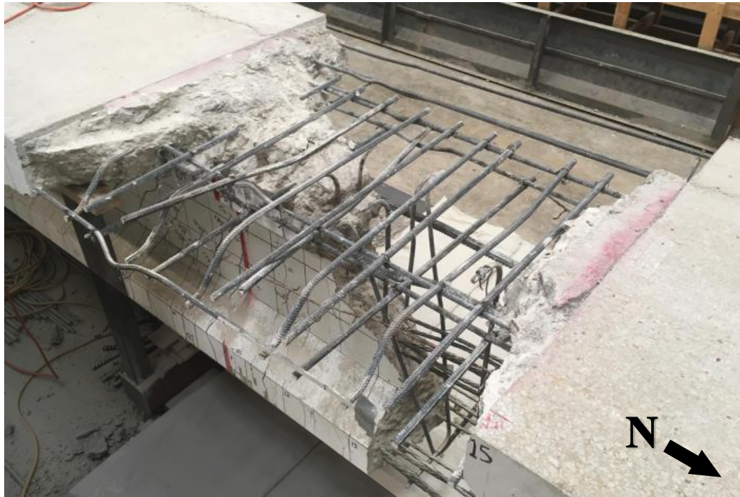
Figure 5.29 Original Deck Reinforcement with Partial Concrete Demo
