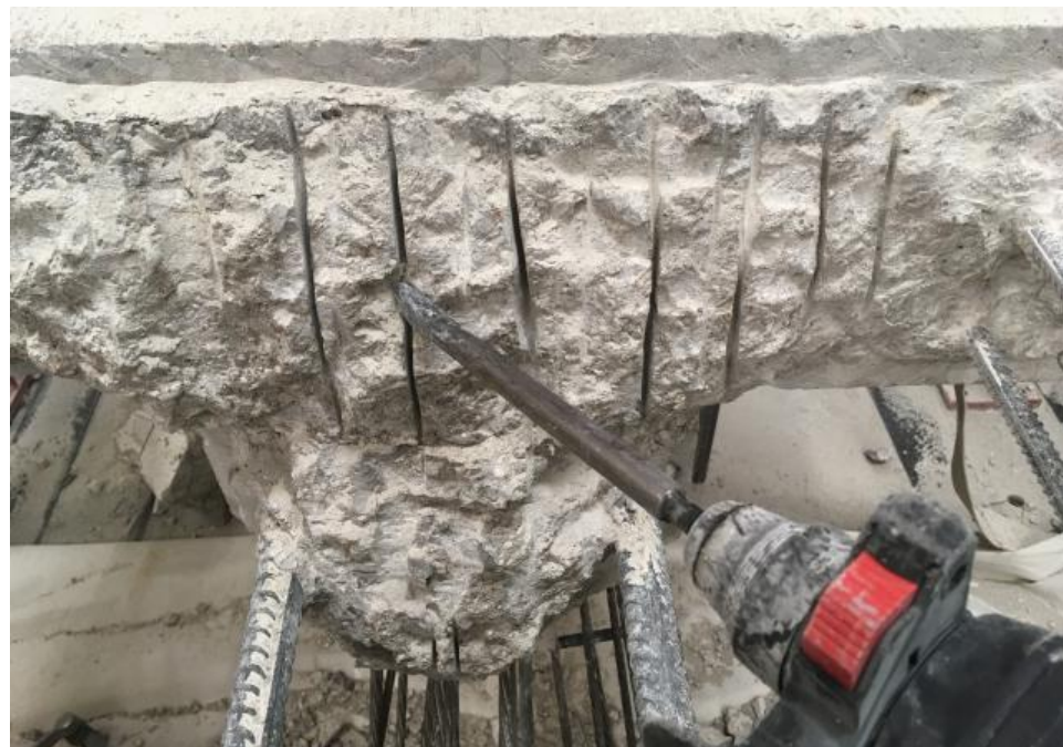
Figure B.4 Removal of Deck Concrete Using an Impact Hammer
