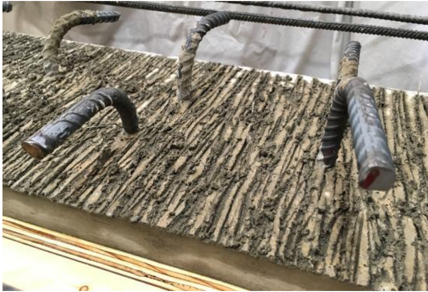
Figure 5.33 Roughened Surface of North End Girder Portion
