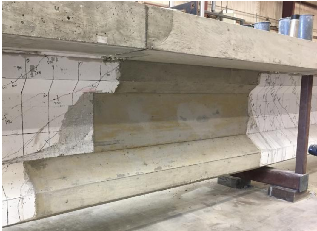
Figure 5.35 West Side of Completed North End Repair
