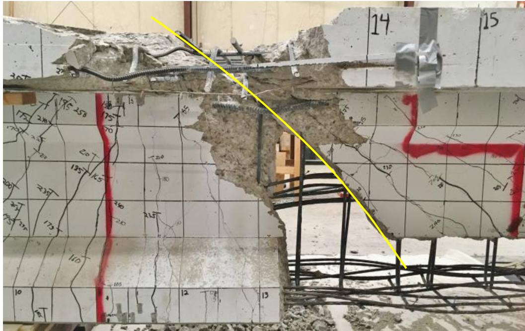
Figure 7.4 North End Shear Plane (Yellow Line) Discovered Mid-Demolition
