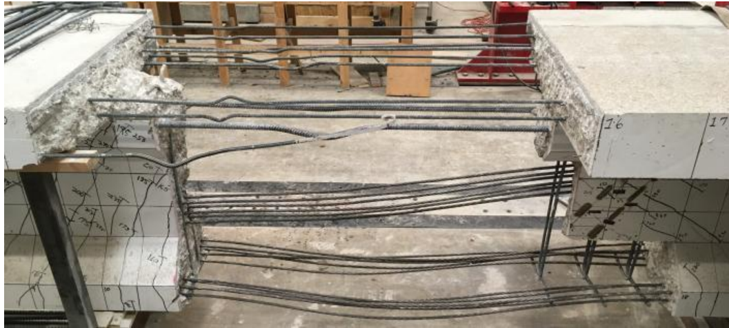
Figure 5.24 North End with Damaged Concrete Removed and Loose, Existing Reinforcing Steel
