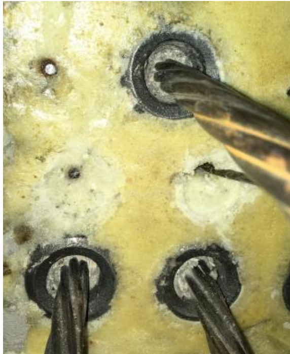
Figure 5.18 Anchor Plates After Casting the South End Repair
