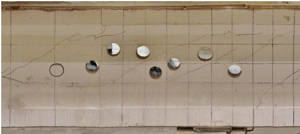
Figure 5.1 West Elevation of Core-Sampled Web Section
