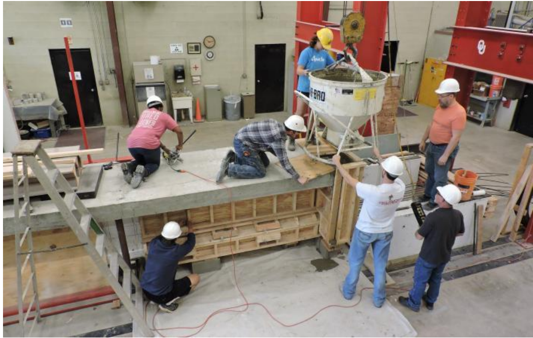
Figure D.3 Adding the FR-SCC Repair Material to the South End
