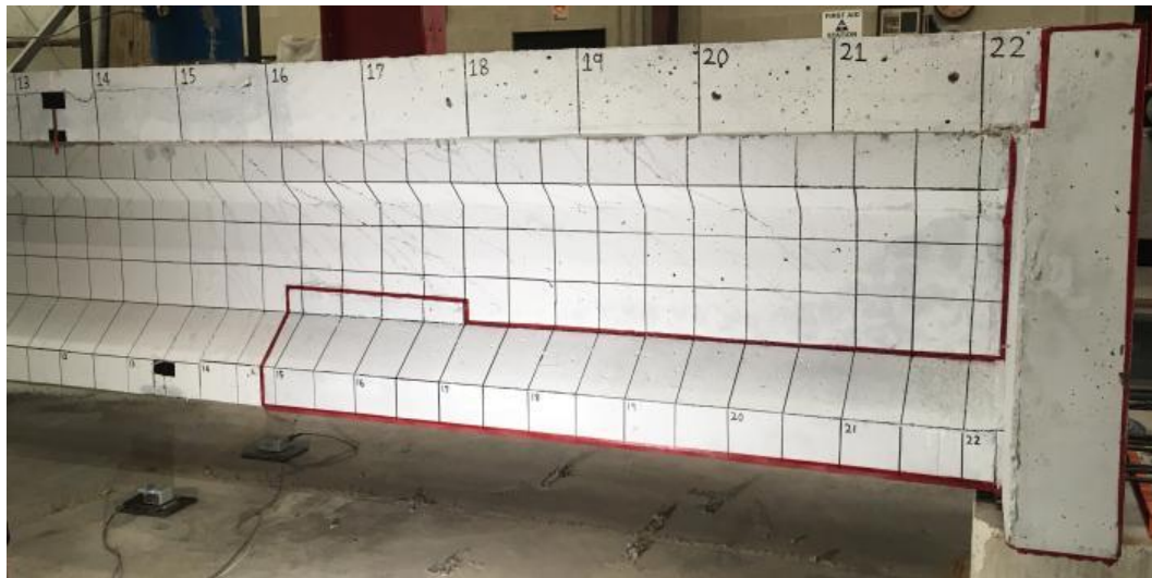
Figure 6.1 South End Repair Section Before Testing
