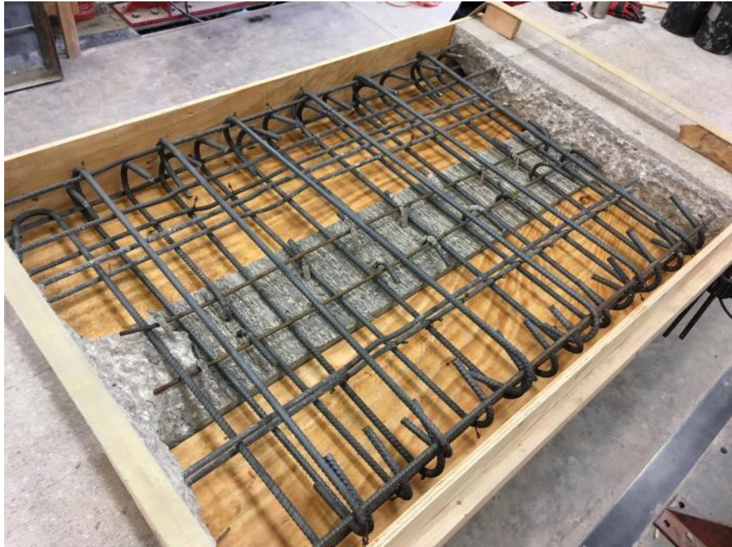
Figure 5.34 Deck Reinforcing of North Repair
