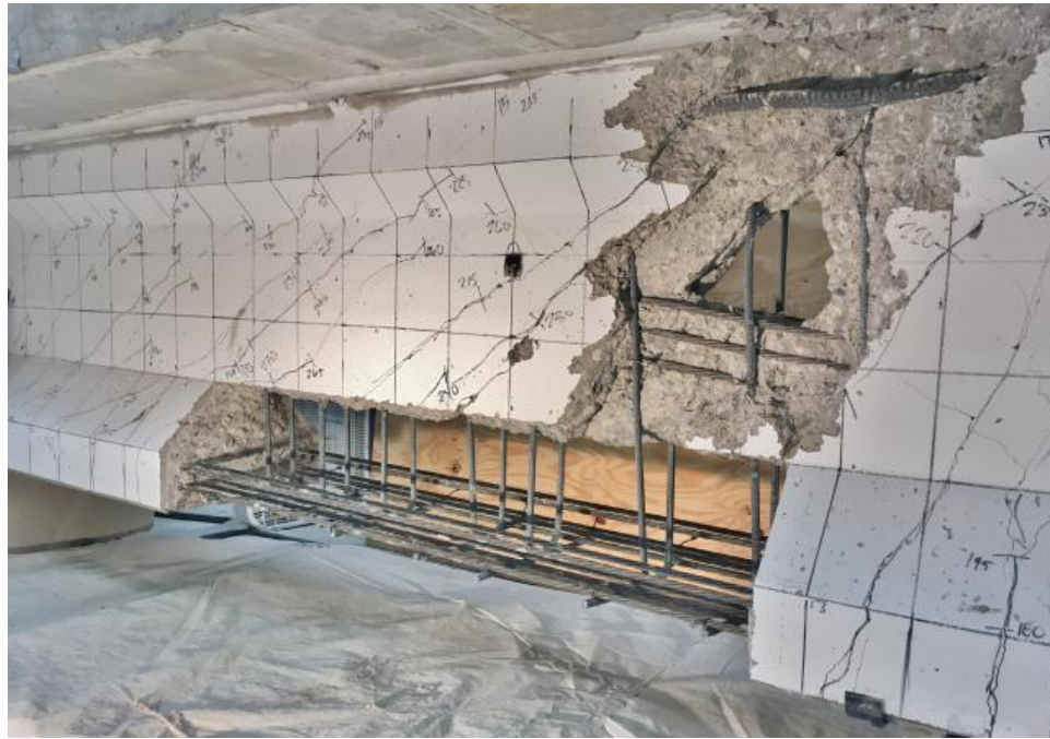
Figure B.3 North End Bottom Bell & Loose Concrete Removal
