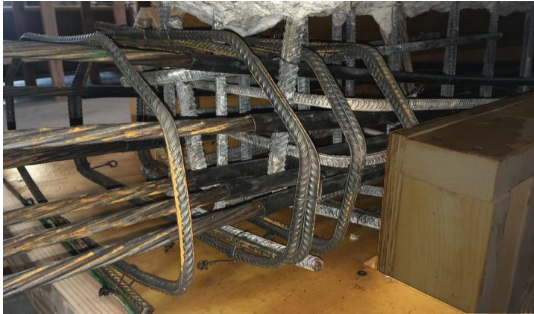
Figure 5.14 Bursting Steel for Post-Tensioning
