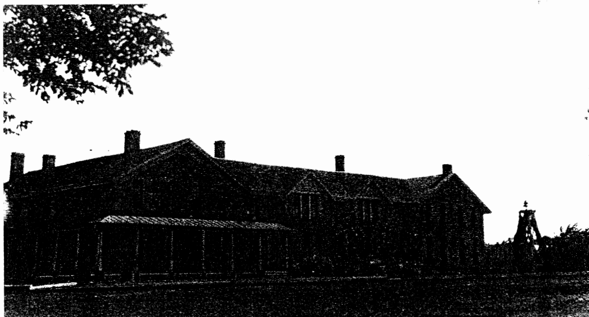
Figure 25. Girls' Dormitory as it appeared after substantial alterations in 1912. Oklahoma Historical Society photograph, negative number 7838.
