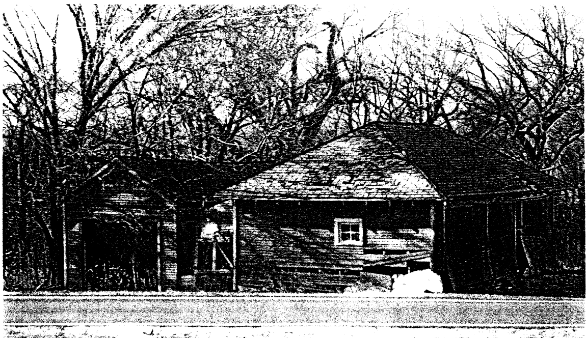
Figure 33. Garages west of the 1909 Principal's Residence, March 2000.
