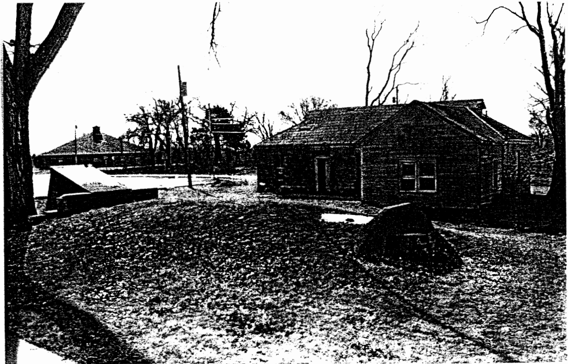
Figure 35. Concrete cellar, with Bakery in the background, March 2000.
