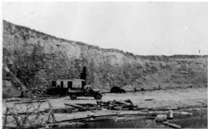
Limestone Face Operating Equipment
