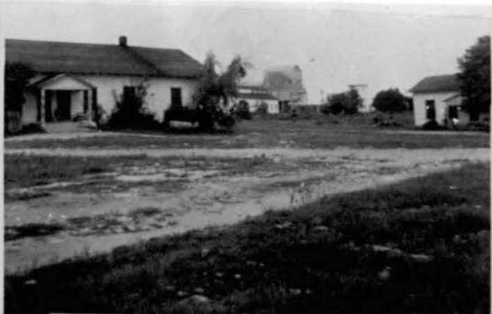
Living Quarters Crusher in Background
