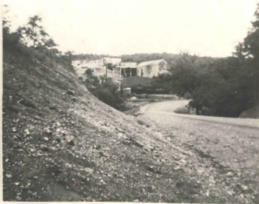
Southern Rock Asphalt Crusher and Mixing Plant
