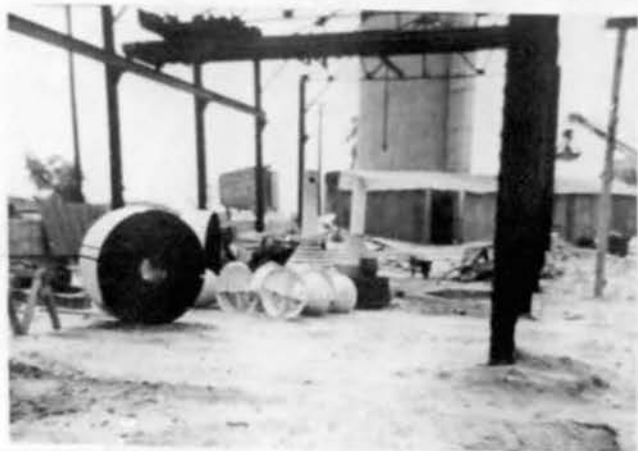
Classifying Baffles Drier in Shed
